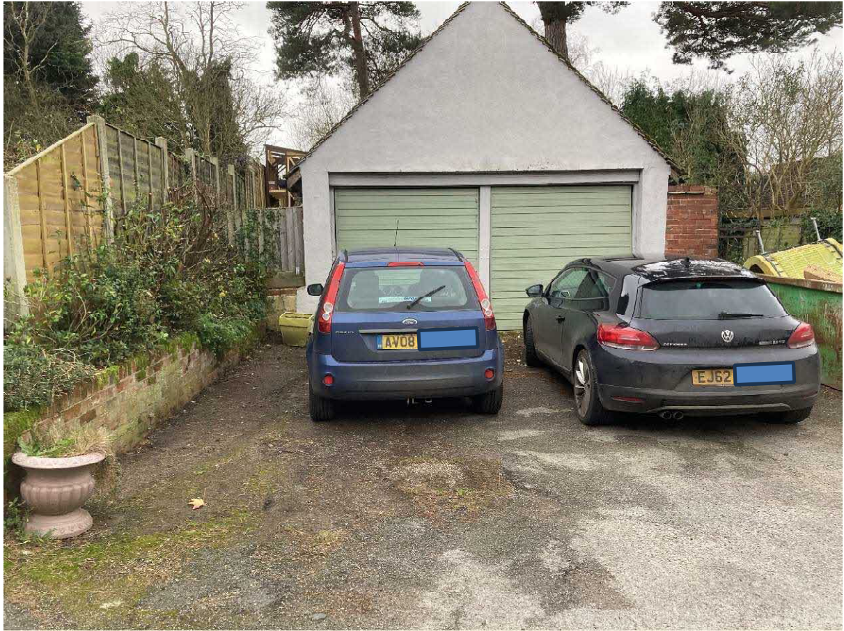
Fig. 7 –View looking south west to LHS of existing garage where new extension is proposed.
