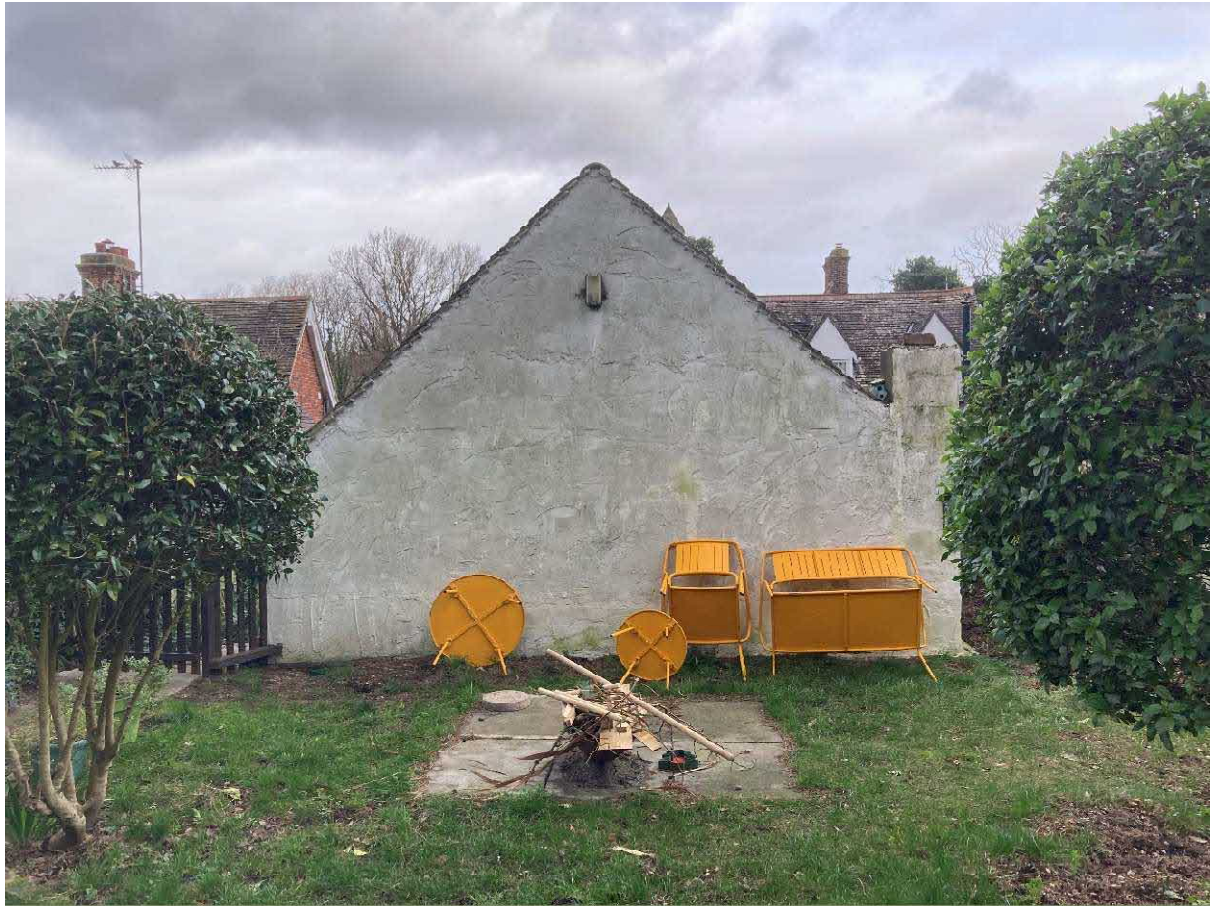
Fig. 10 –View looking north east towards The Bell House. Note chimney to RHS of gable wall
