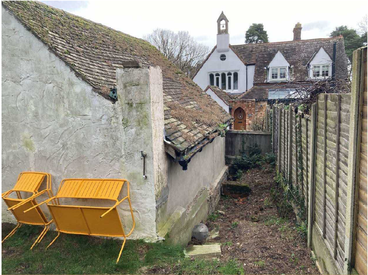
Fig. 11 –View looking north east towards The Bell House. Change in ground levels can be seen, as can the retaining wall/DPC level. Area to RHS will house the proposed+
