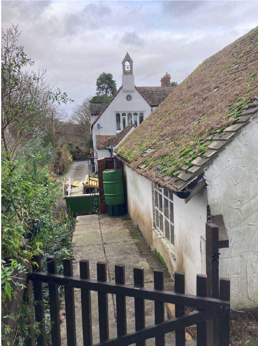
Fig. 9 –View looking north east towards The Bell House with the existing garage immediately to the RHS
