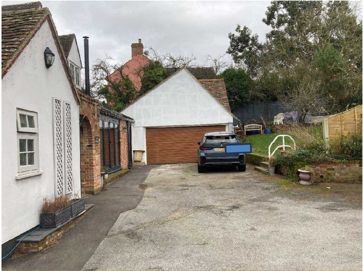
Fig. 5 –View looking east, 'The Bell House' to LHS with converted garage to front. Note rear facing dormer.
