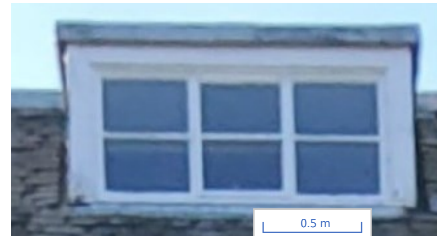
Detail: Steel Frame Attic Dormer Window
