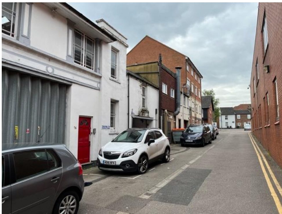
Varying roof heights on Stuart Place, behind the application site
