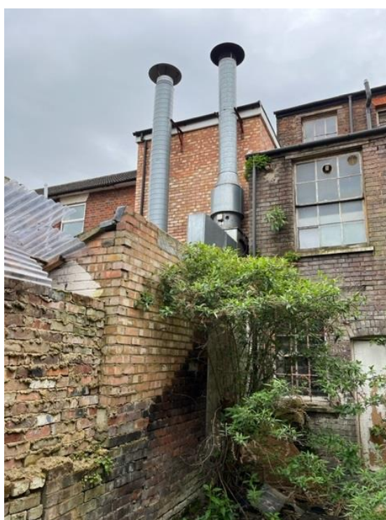
Rear extension at 72 Wellington Street
