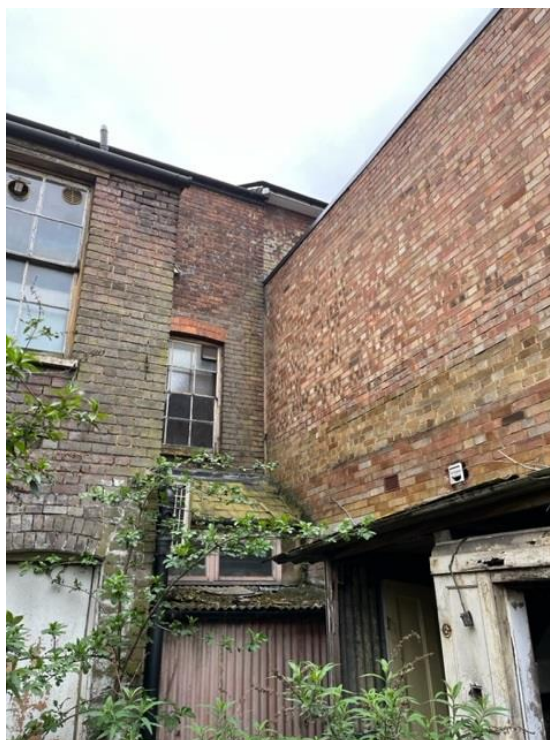
Rear extension at 76 Wellington Street
