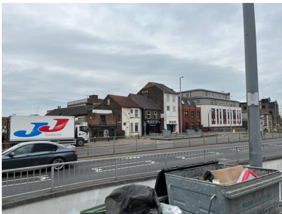
Varying roof heights on Stuart Street, opposite the application site
