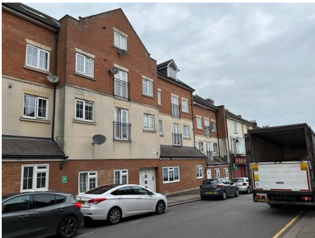
Four storey flats on the west side of Wellington Street
