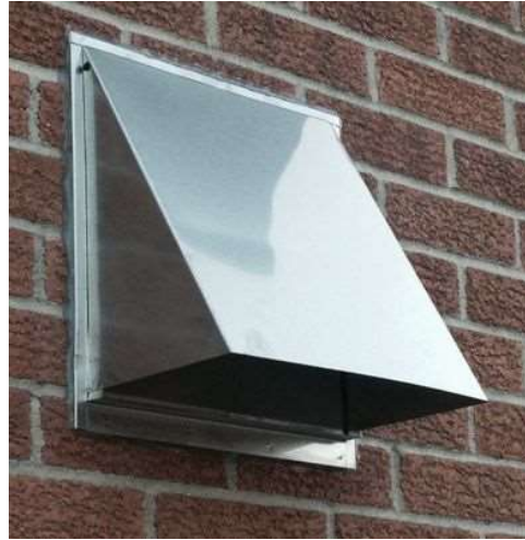
Kitchen Extract Fan Flue
