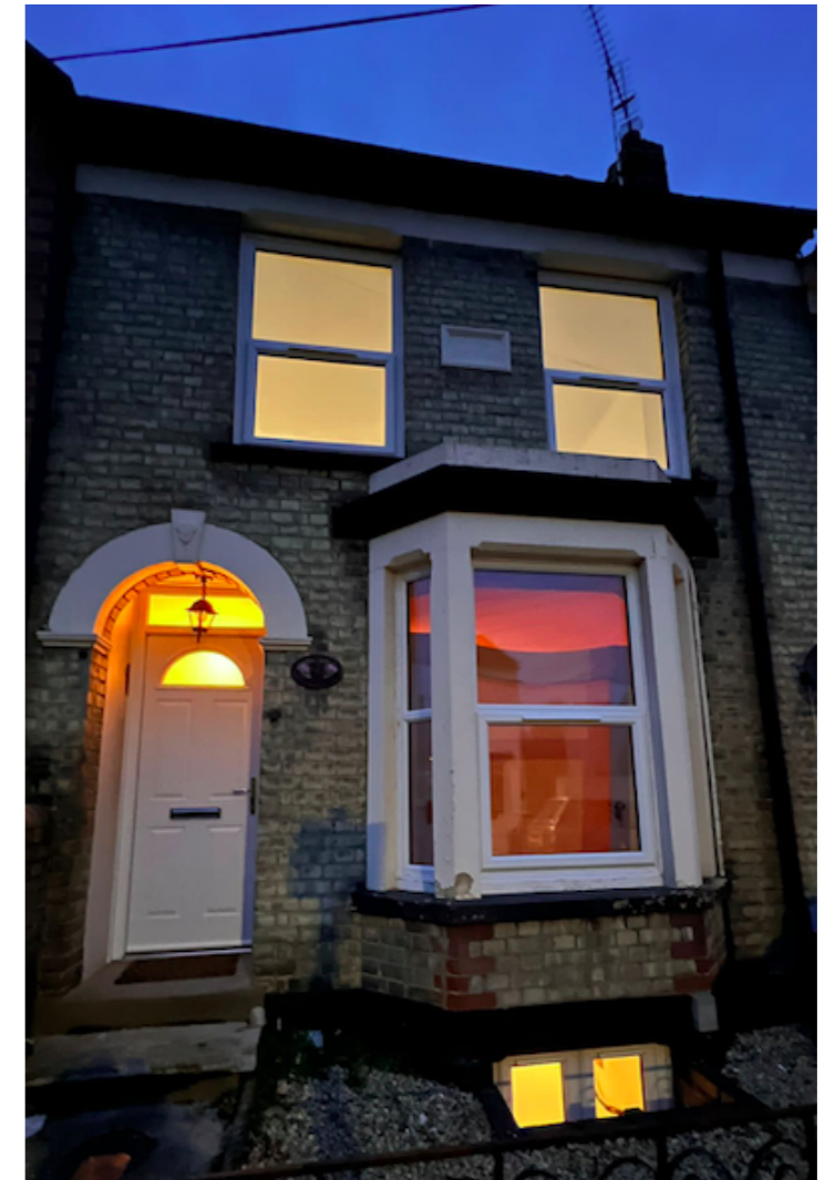
PHOTOGRAPH: EXISTING FRONT ELEVATION
