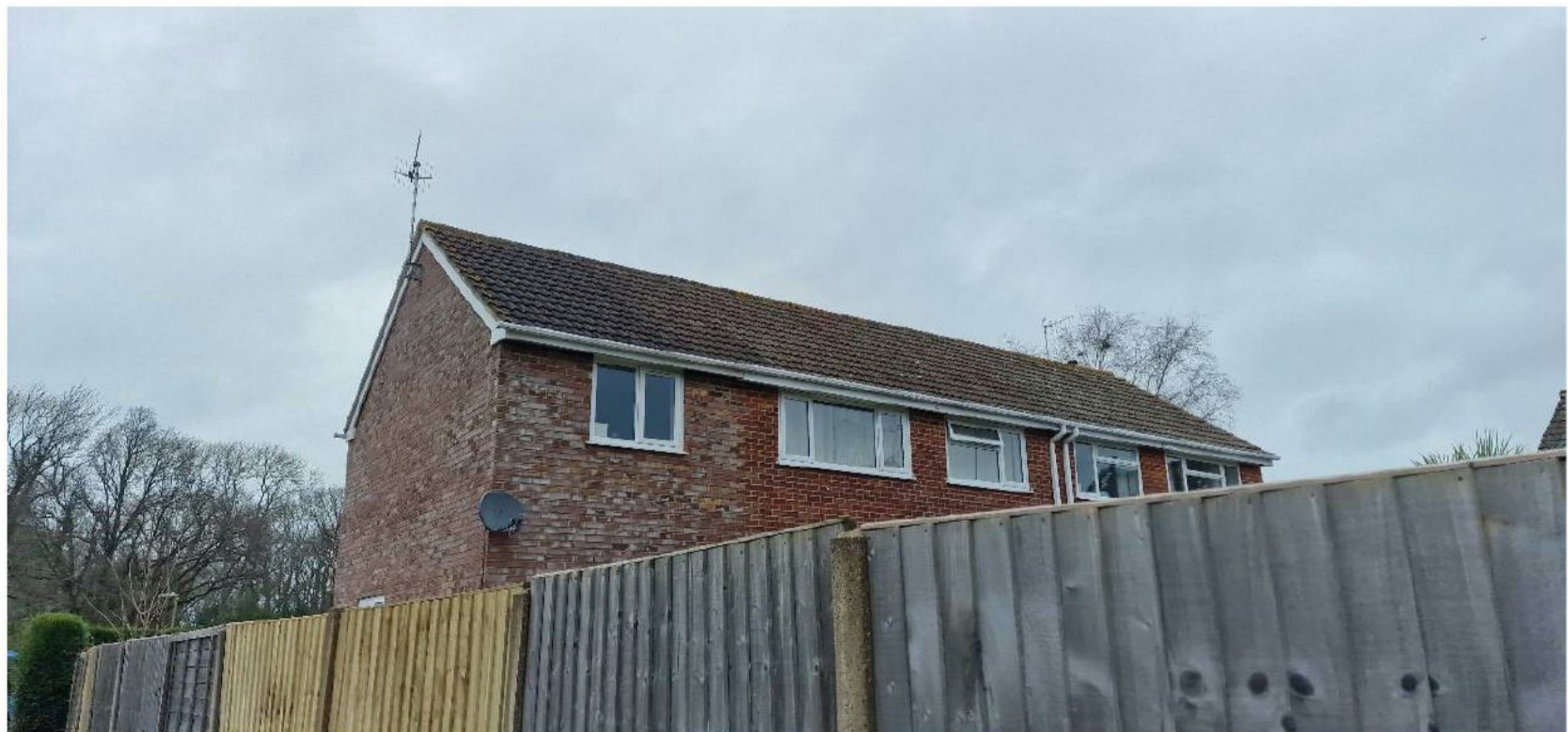
Picture 2: Showing the rear elevation
