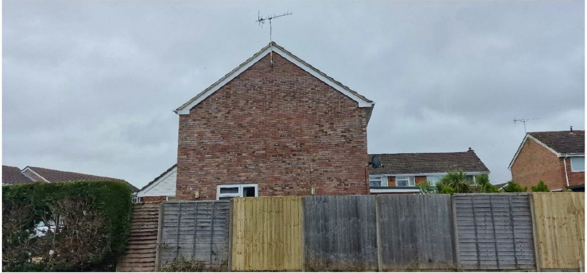
Picture 3: Showing the side of the building.
