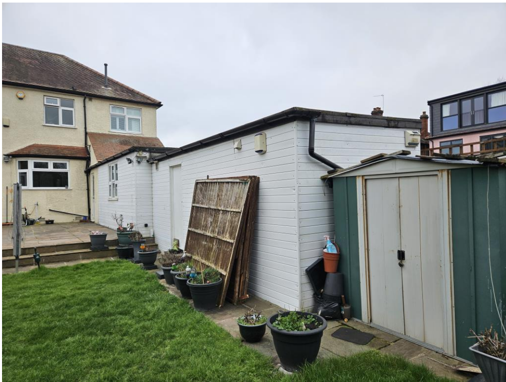
4. Rear view towards communal driveway
