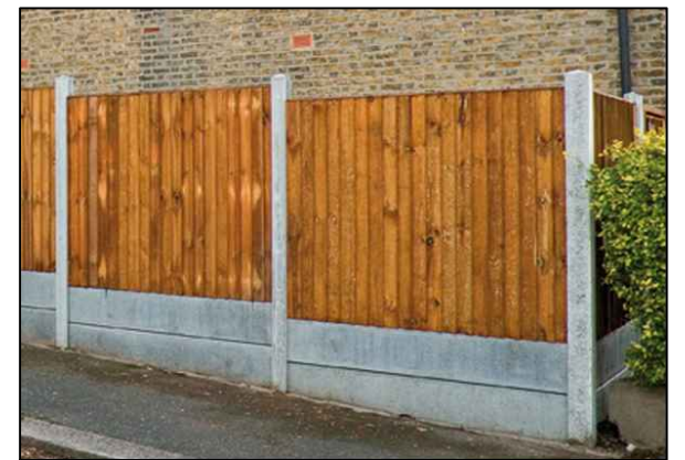
Close Boarded Timber Fencing with Concrete Gravel Boards and Posts.
