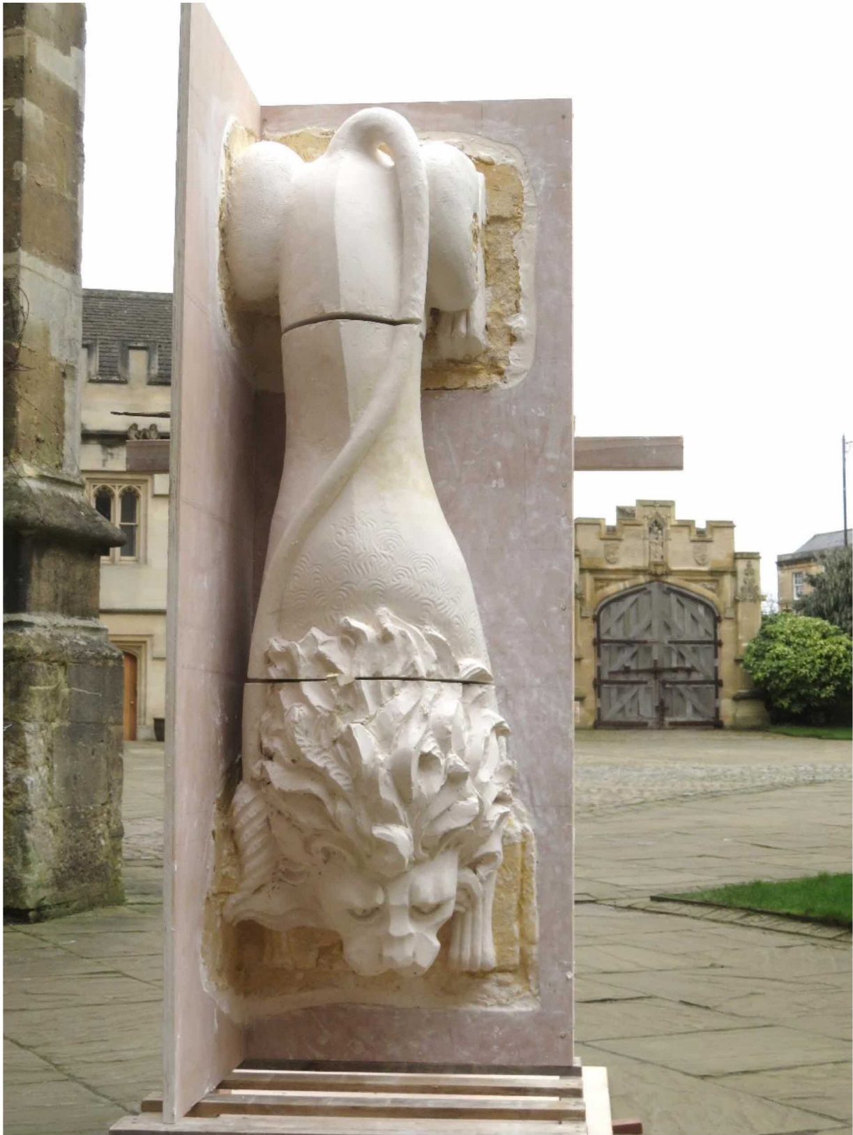
Fig 27: front elevation of model, showing joint position and tufted tail tip
