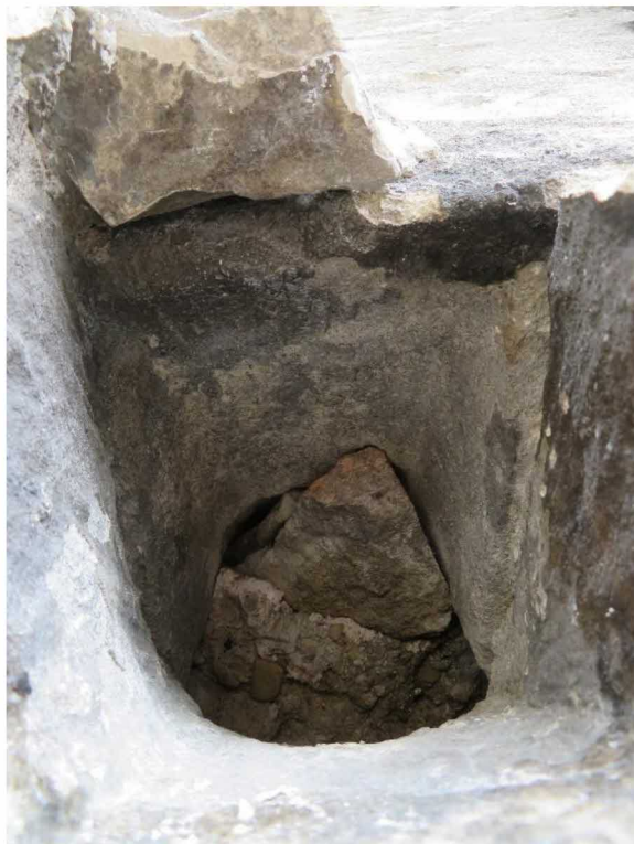
Fig 10: interior of hole capped off
