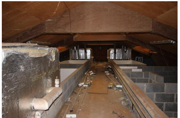
6. Roof space above central corridor
