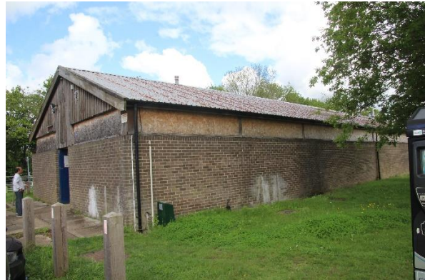
2. Building from the south-east
