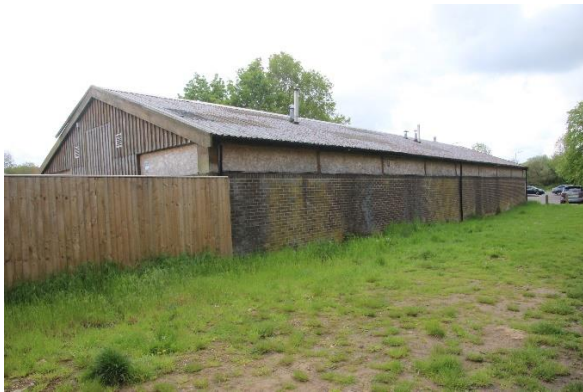
1. Building from the north-west
