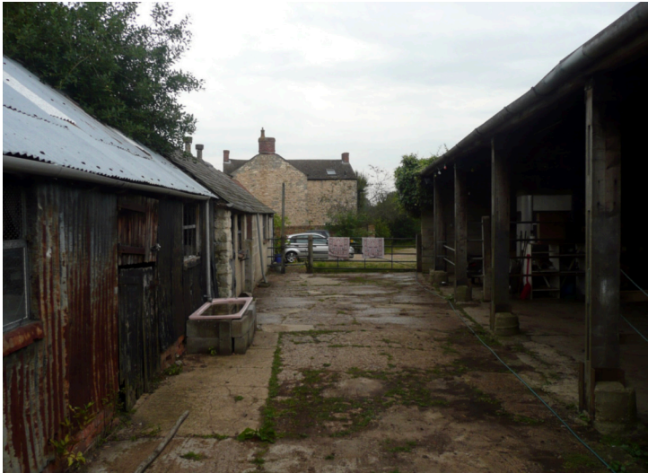
Photo of old farm yard pre demolition
