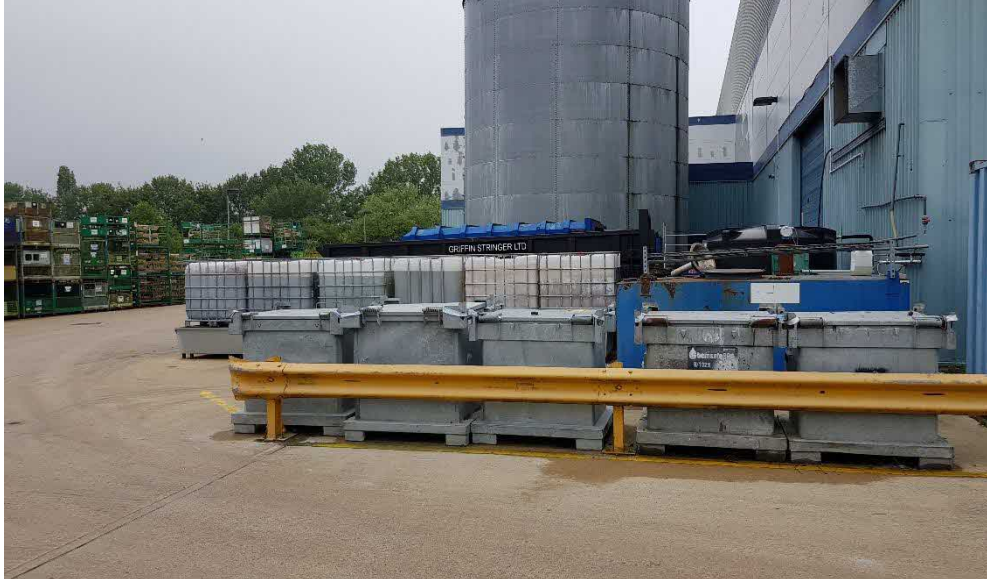
Photo 5: 5no. steel storage containers with IBC's and Storage tank, facing NW
