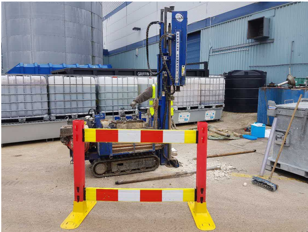
Photo 12: Window Sampler rig at BH4
