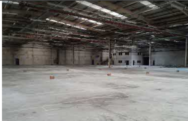
Figure 9 - View of internals of building 1.
