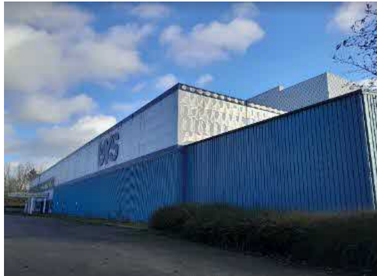
Figure 8 - View of western face of building 1.
