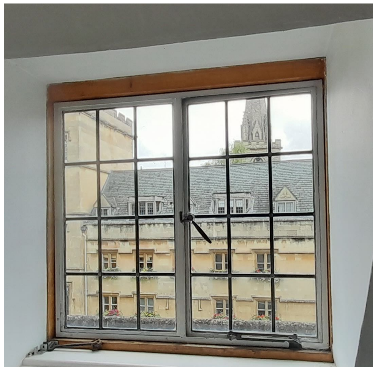
Existing Window MC-1
