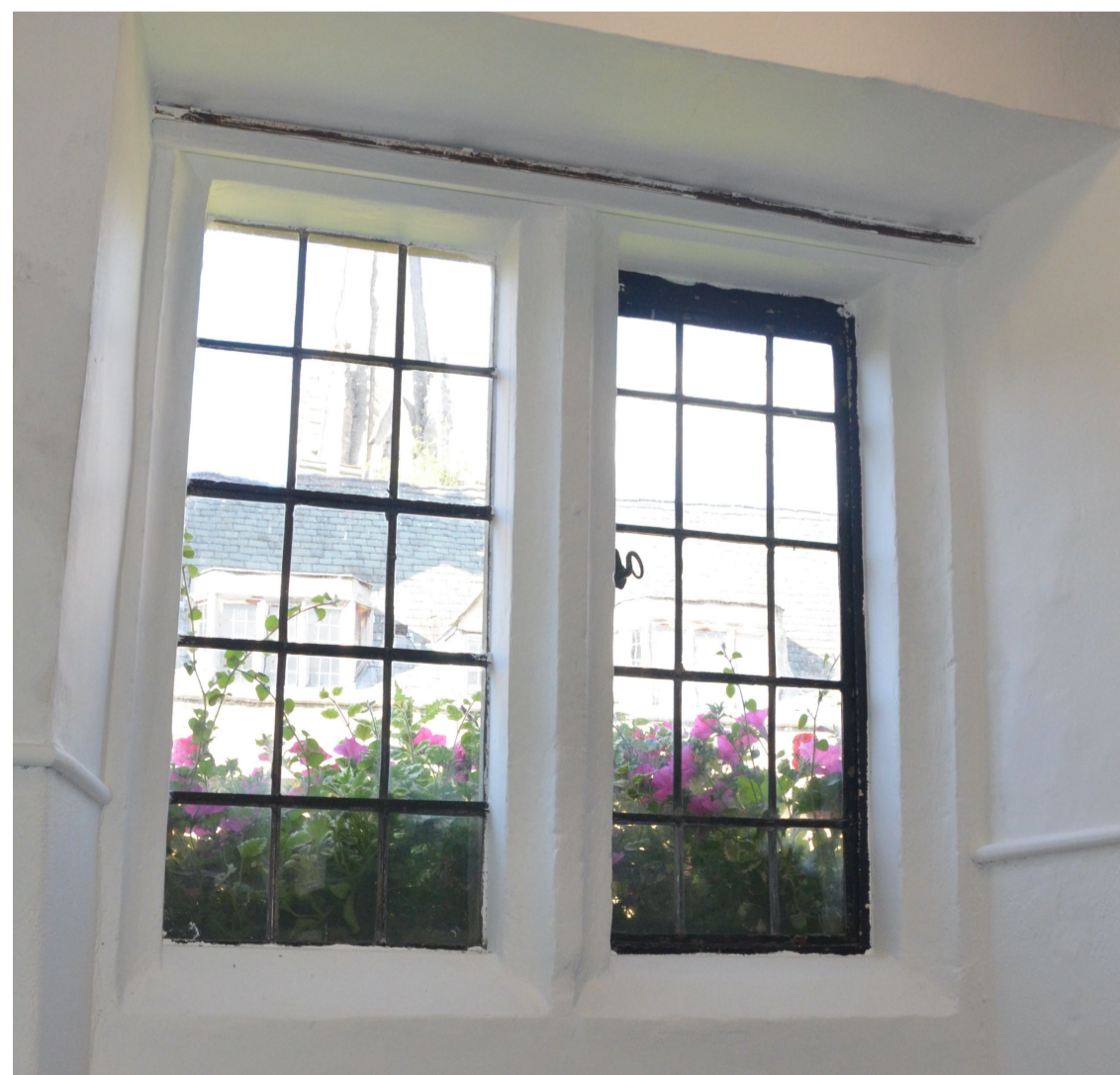
Existing Window S-1
