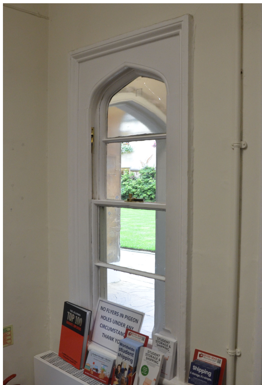
Existing Window TS-13
