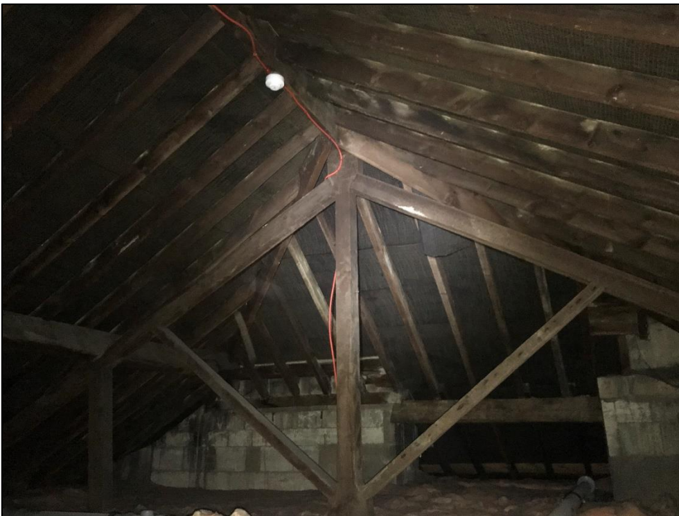
Figure 6: Internal loft void within B2/SC8
