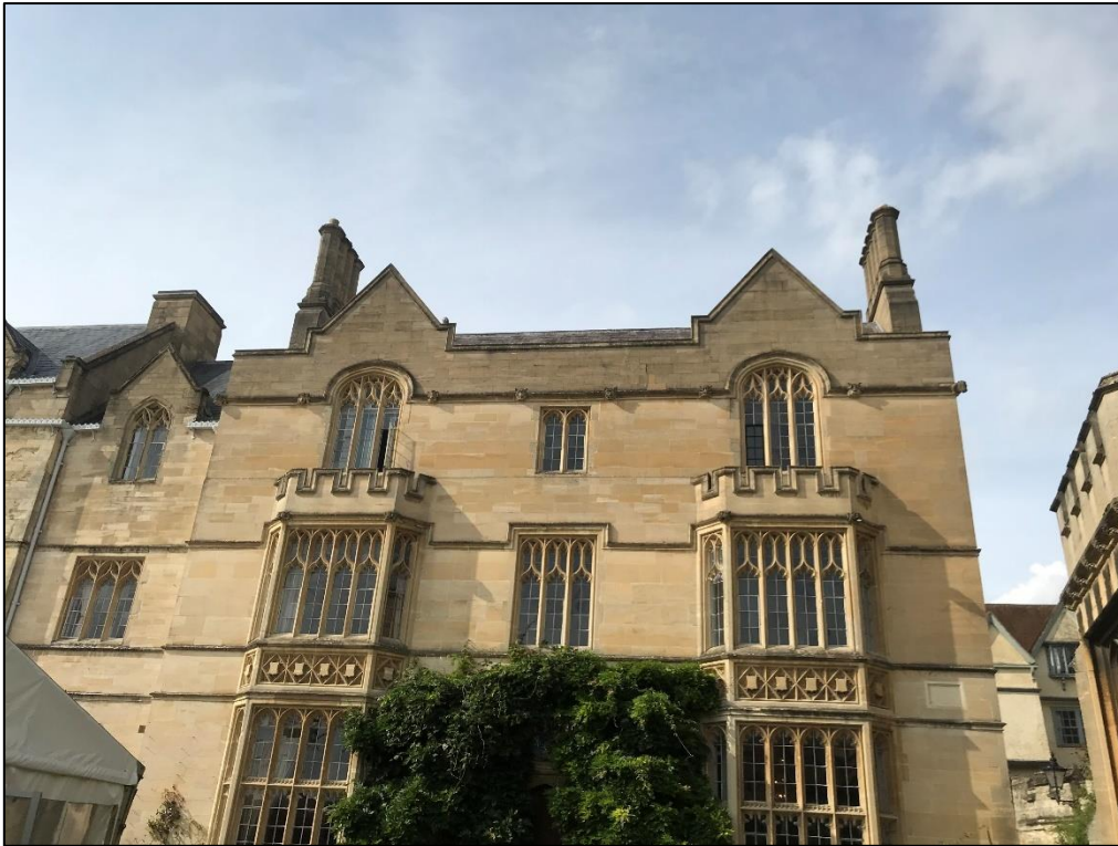
Figure 4: B1/SCR located to the north of Chapel Quad
