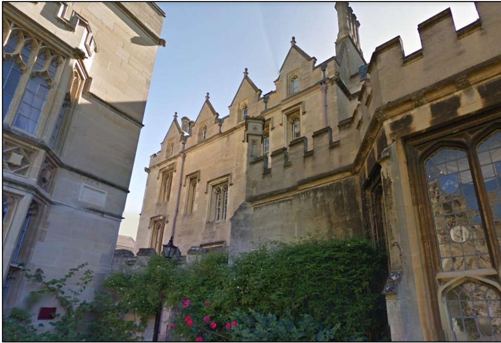
Figure 5: B2/SC8 located to the north-east of Chapel Quad
