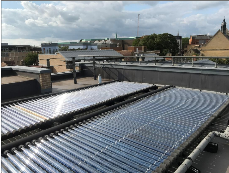
Figure 8: Roof top of one of the buildings within ROKOS Quad
