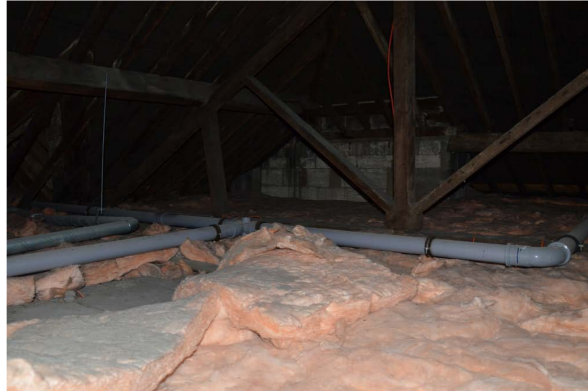
Loft of Staircase 8
