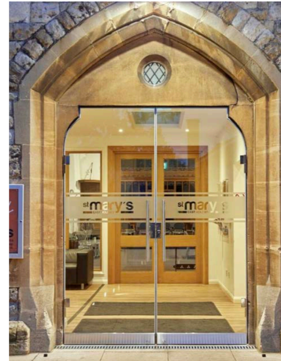
Examples of Ion Glass frameless glass doors within historic openings St Mary's Church, Molesey
