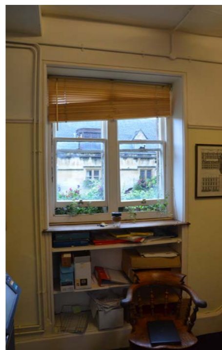
Examples of windows with the same general configuration but different sill conditions. Also note the window shades, which will clash with secondary glazing positions
