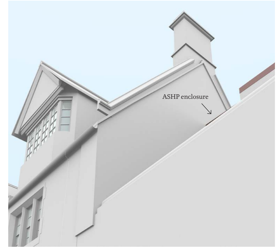
View 02 – Small glimpse of ASHP enclosure from Brewer Street
