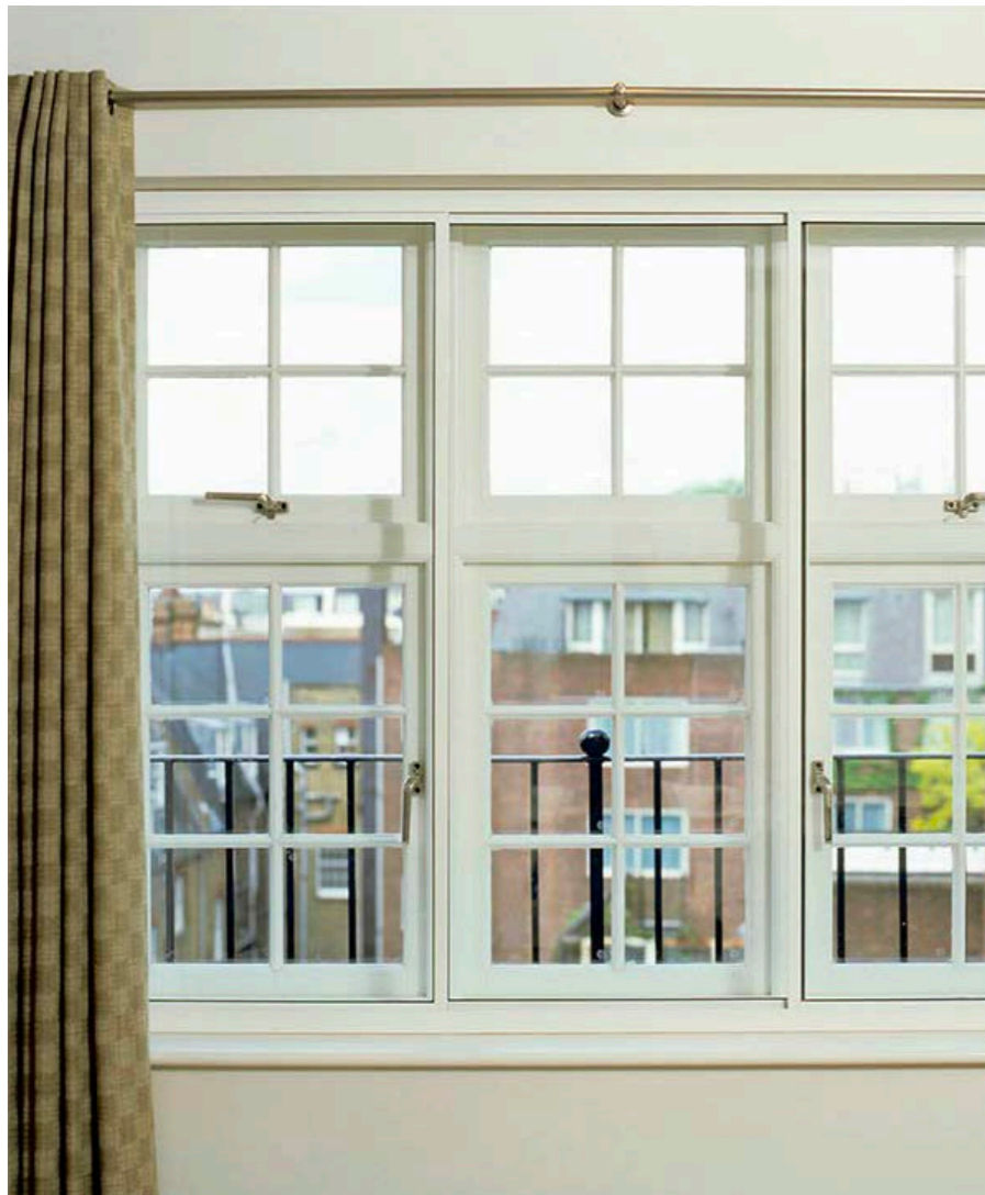
Example of Selectaglaze horizontal sliding system applied to multi-part sash window
