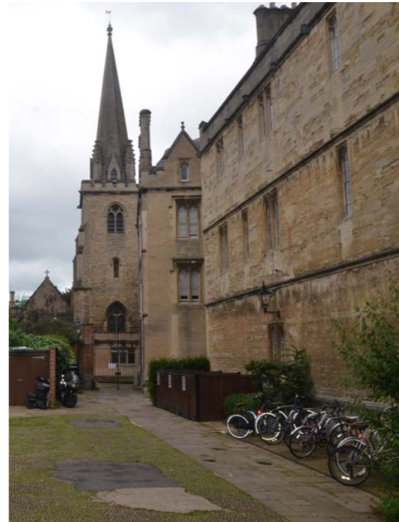
North wall of the SCR Staircase
