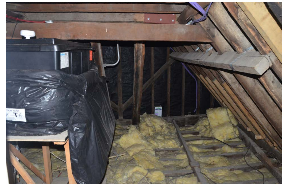
Loft of lower roof area in Tower Staircase (above T.07)
