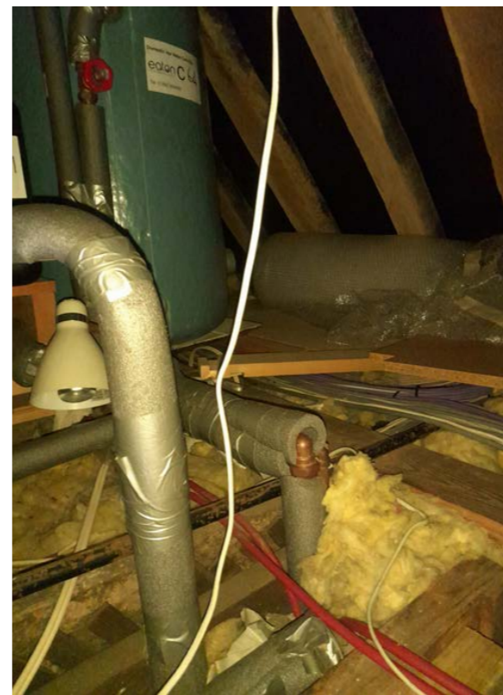
Loft of Staircase 4
