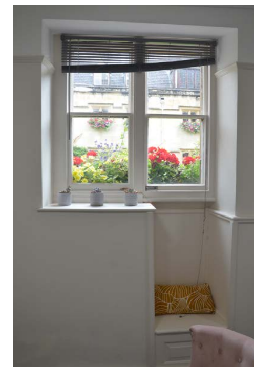
Examples of windows with the same general configuration but different sill conditions. Also note the window shades, which will clash with secondary glazing positions
