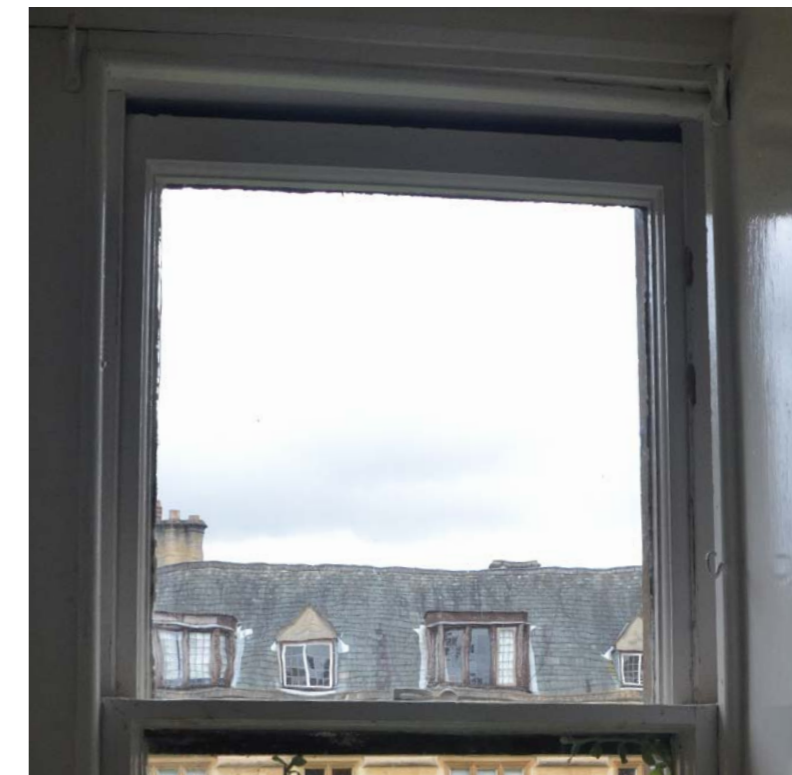
Window with cylinder glass (note the 'wobbly' effect)
