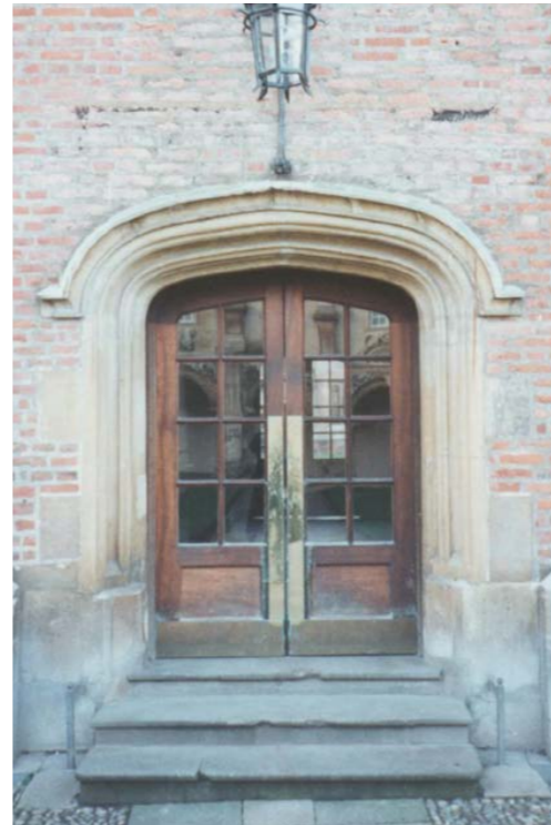
Modern timber door within a historic opening Magdalene College, Cambridge
