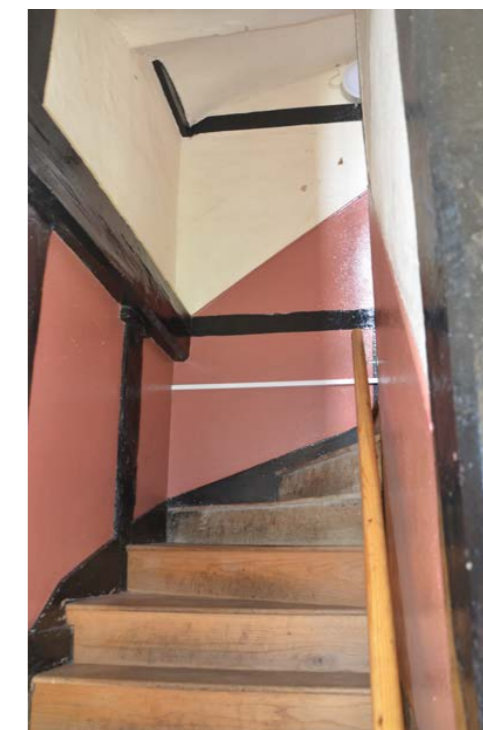
Staircase 3 - black beams and bold colours
