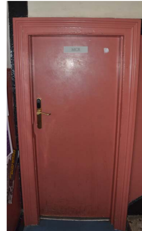
Modern flush door in Staircase 3
