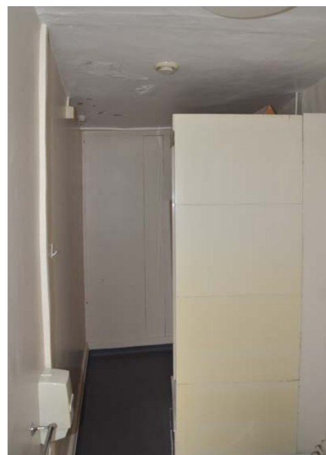
Dead space within bathroom of room 7.3
