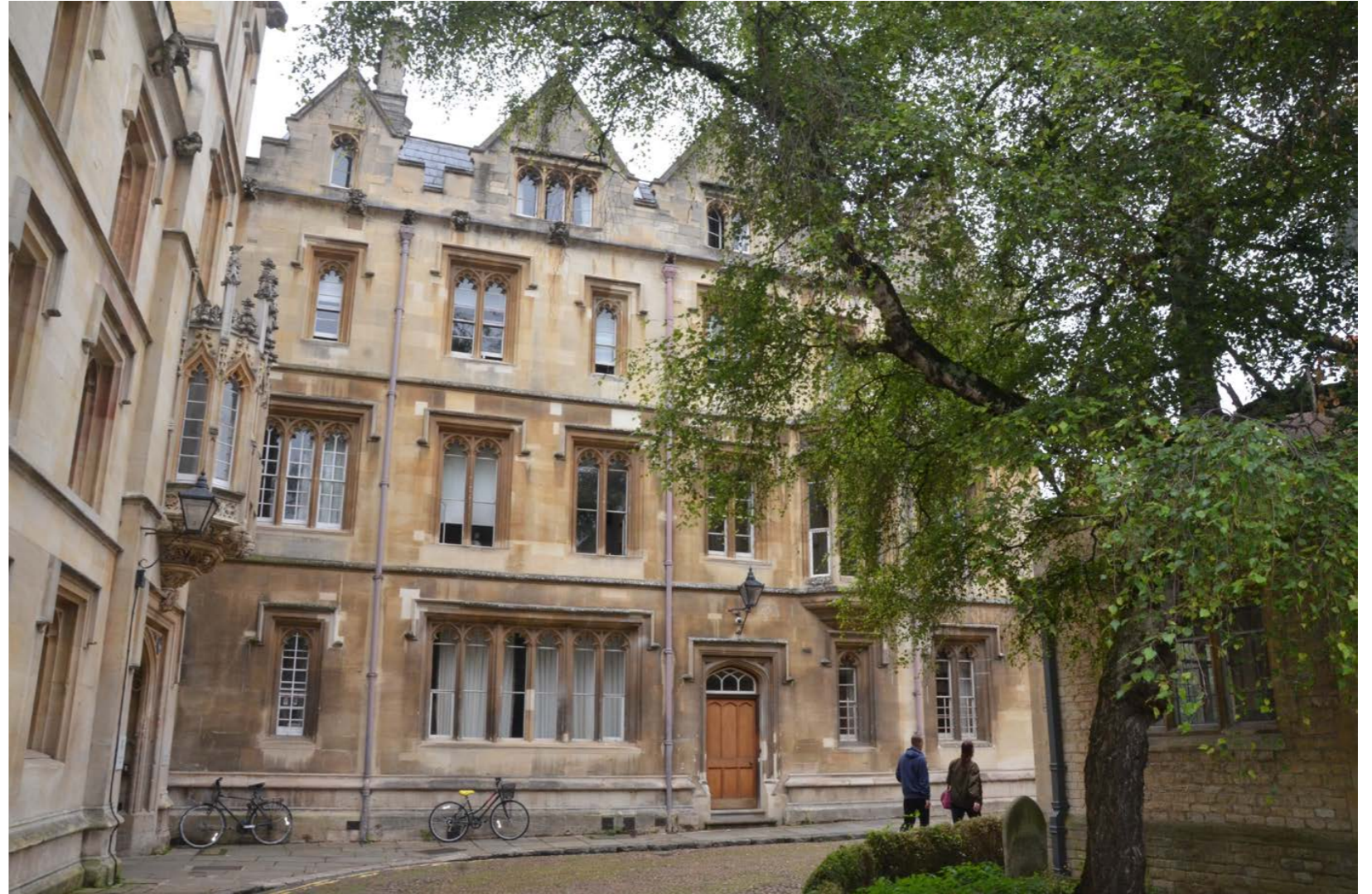
East elevation of Staircase 8
