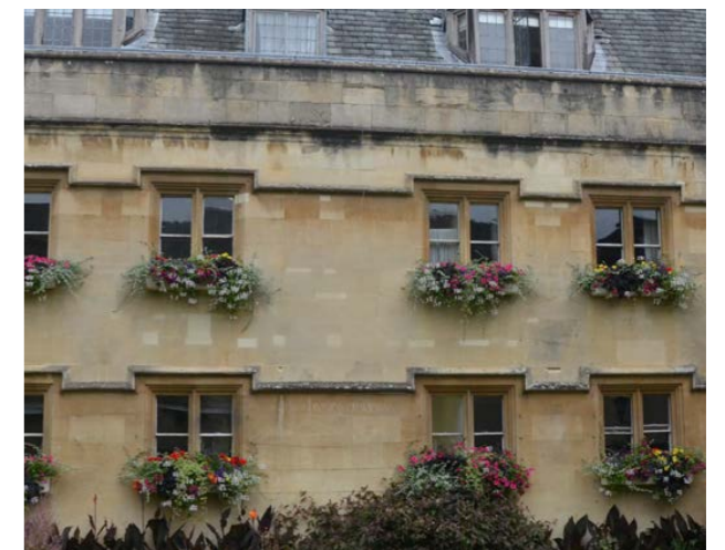
Patch repairs to stonework
