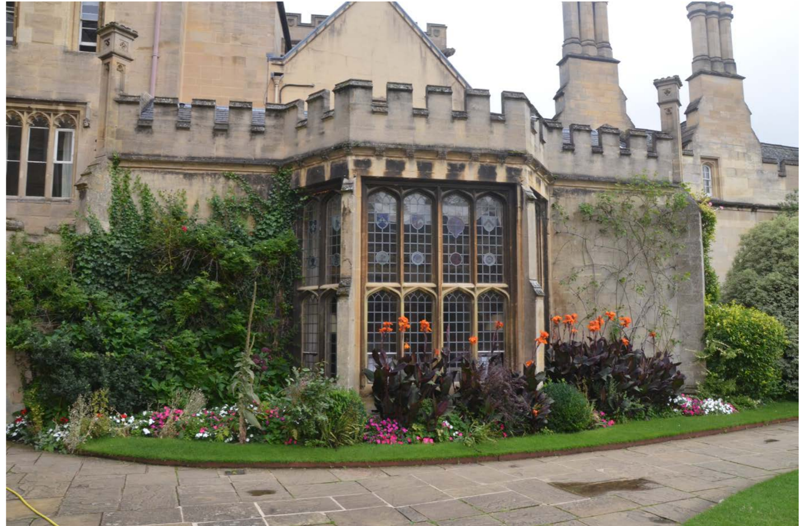
West elevation of Broadgates Hall
