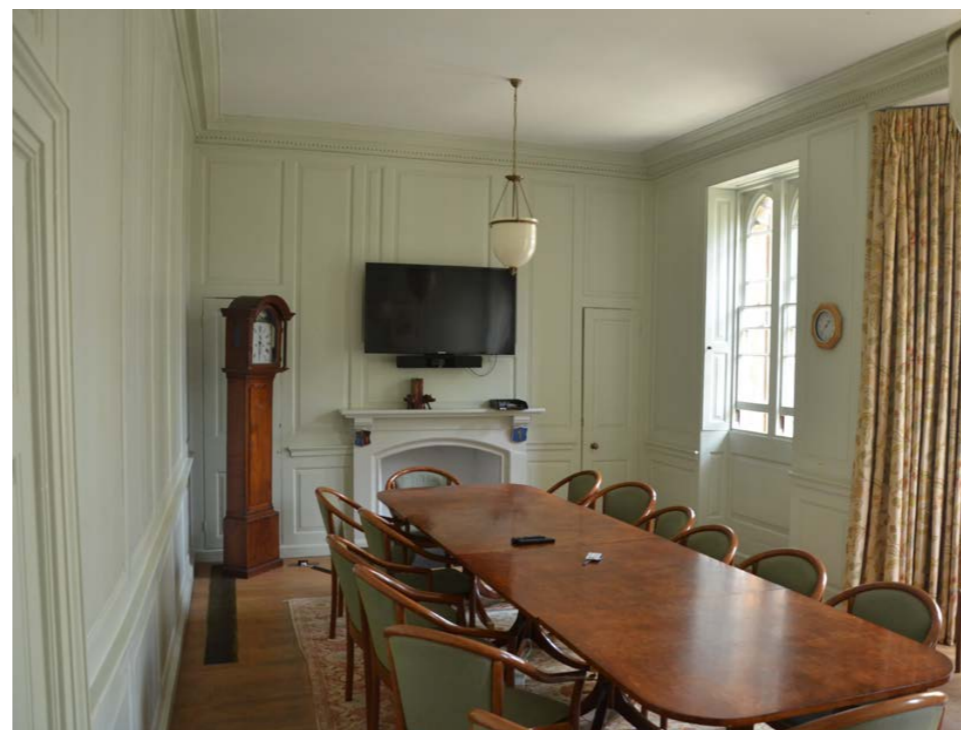
Timber panelling in room 8.23
