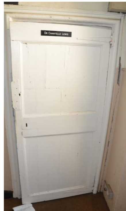
Outer leaf of double door in Staircase 4
