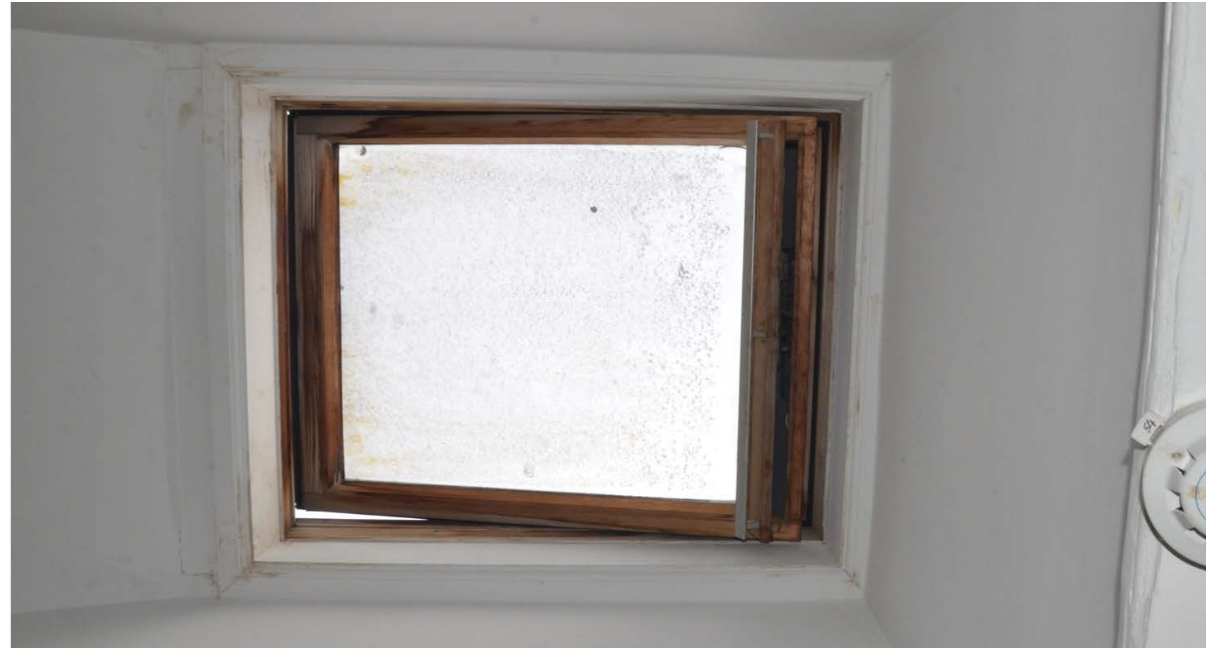
Rooflight Type 1 within Staircase 8 circulation
