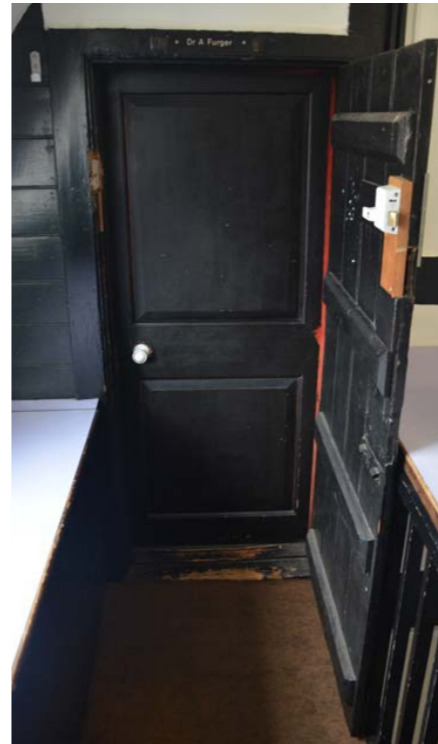
Double door within Staircase 5
