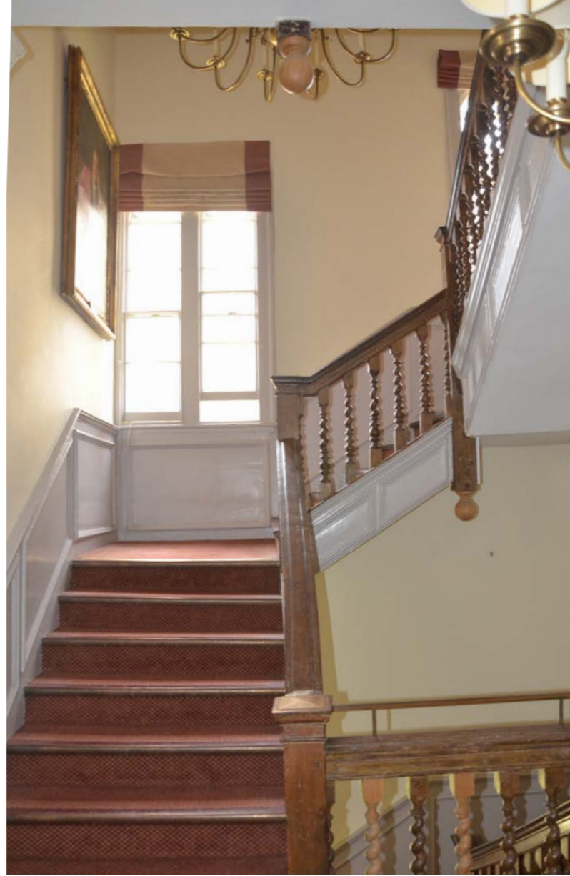
Staircase 8 circulation – first floor level
