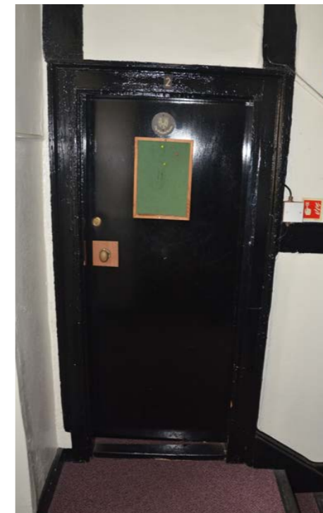
Modern flush door in Staircase 7
