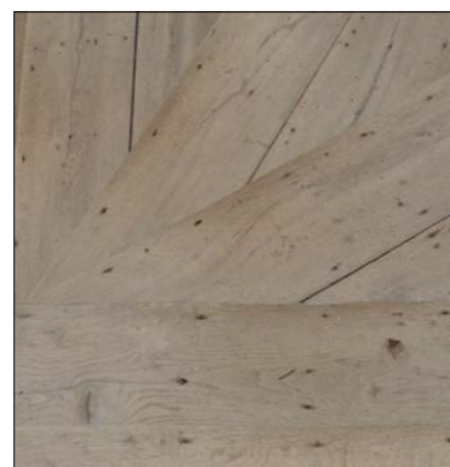
Exposed timber boards to floor in Staircase 7
