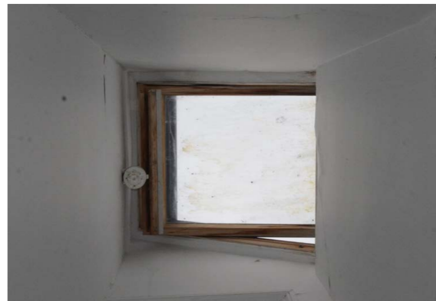
Rooflight Type 1 within Staircase 8 circulation
