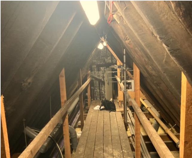
Photograph 10: Timber roof structure above Staircase 2
