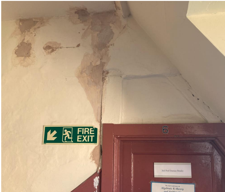
Photograph 5: Remedial works on 2nd floor landing of Staircase 3
