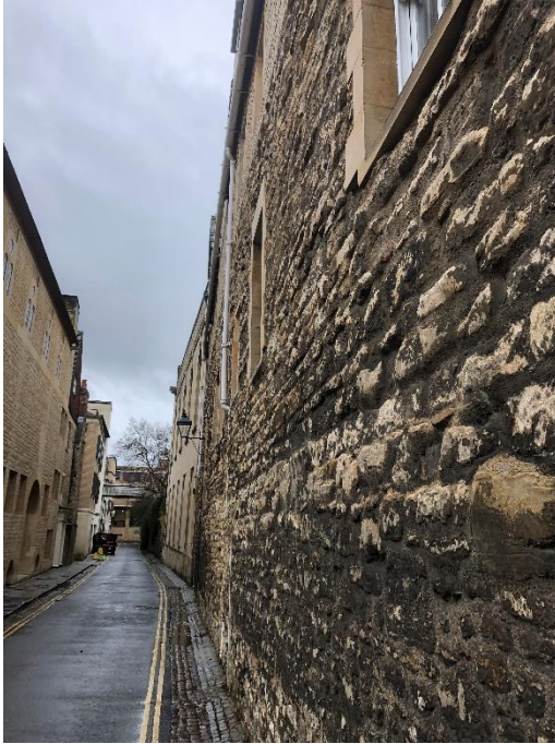
Photograph 18: External Wall Brewer Street
