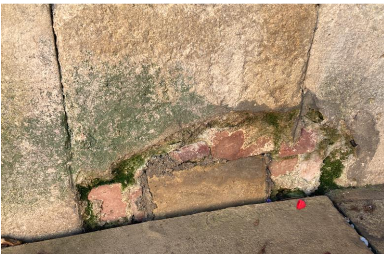
Photograph 28: Remedial works to stonework now with algae/moss
