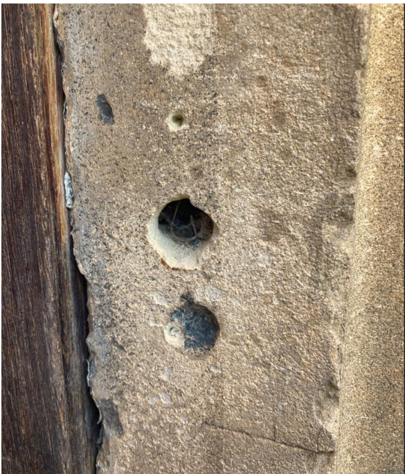
Photograph 25: Stonework next to entrance of Staircase 2
