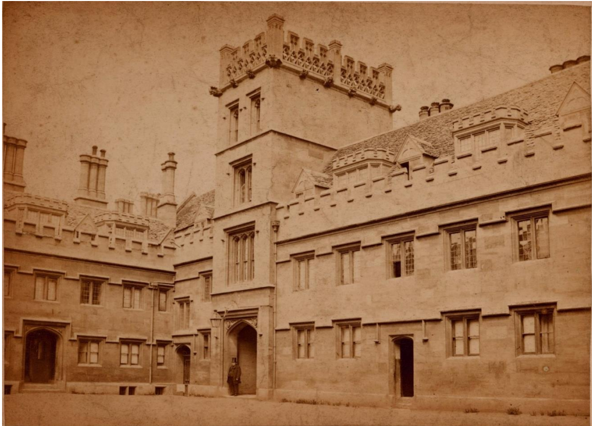
circa 1870-72: North range, South elevation & West range, East elevation (Pembroke College Archives)
