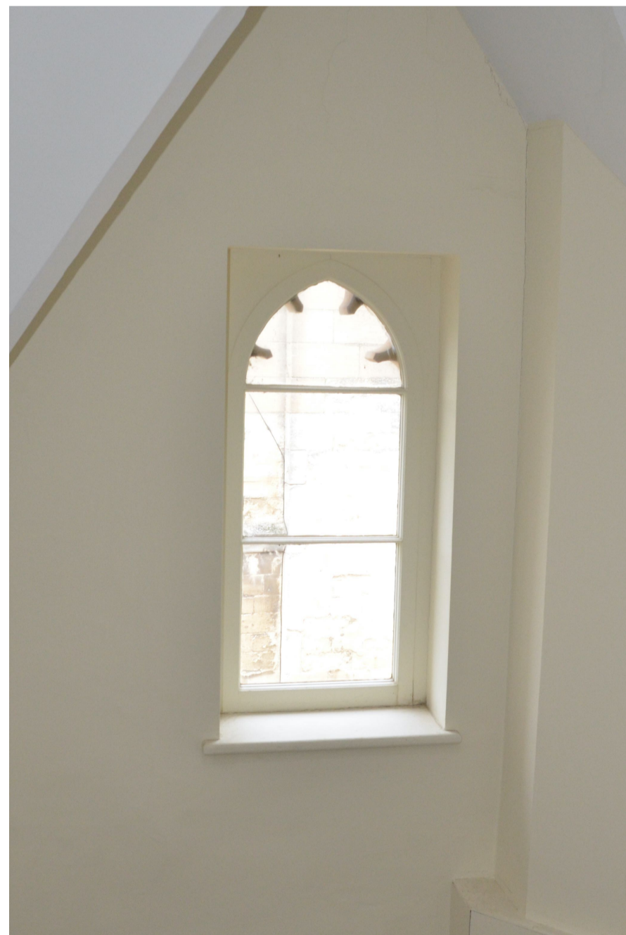
Existing Window TF-1
