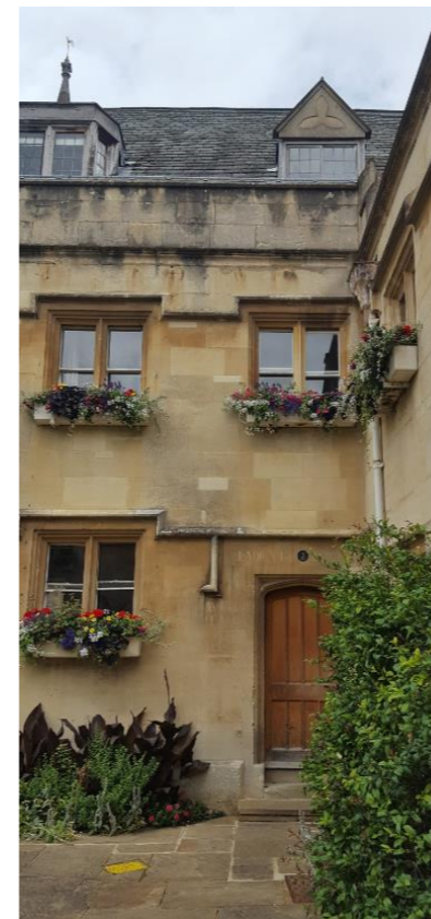
Precedent recent addition of a door to Staircase-2
