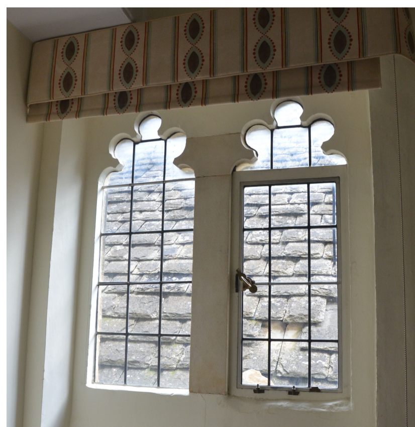
Existing Window S-6
