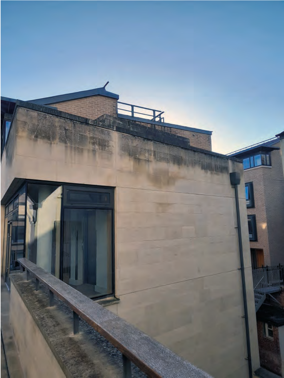
Plate 12: Rooftop on Rokos Quad, view looking south
