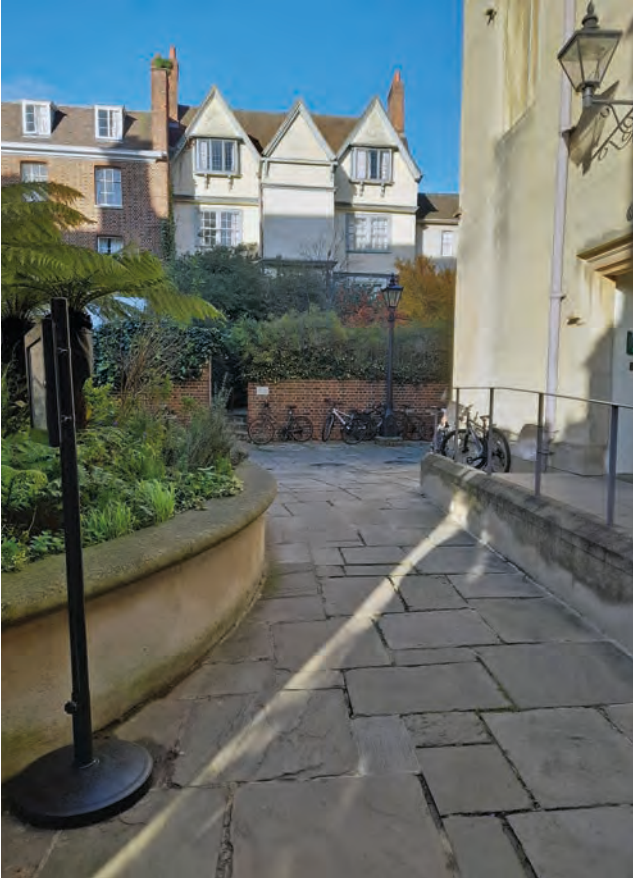
Plate 8: Cabling route along the western wall of the Old Quad, view looking north
