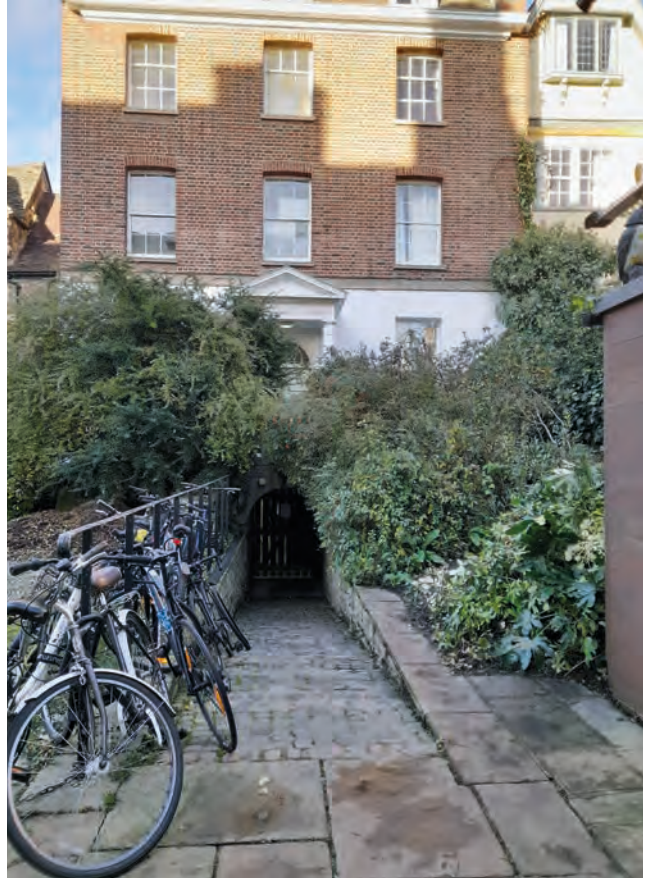
Plate 9: Ground in front of Staircase 17, view looking north
