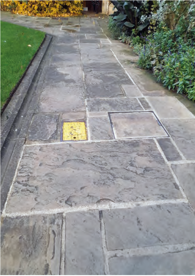
Plate 3: Traces of existing cabling trenches within the Old Quad
