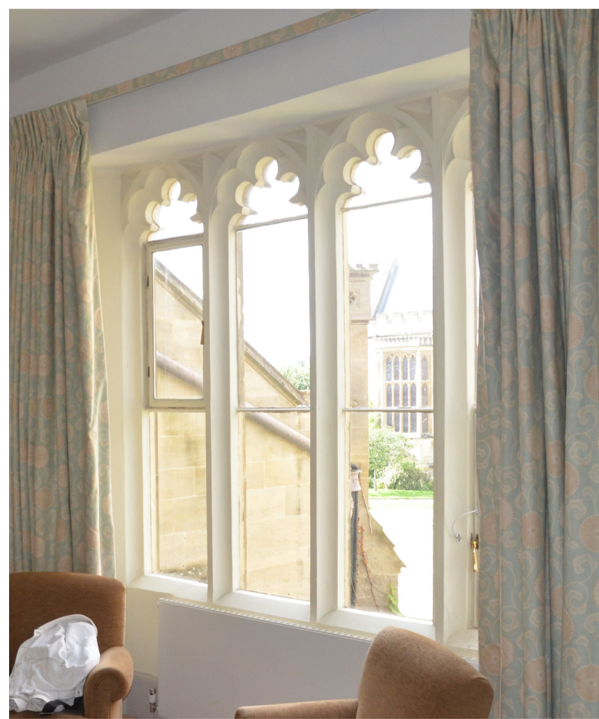
Existing Window S-5
