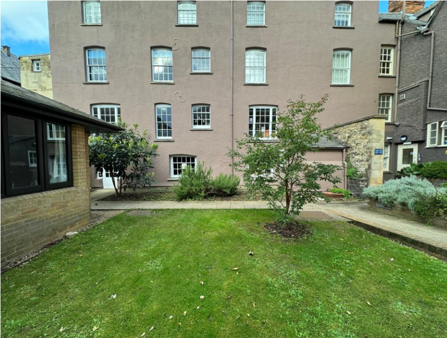
Image 01 – South elevation of no 1 brewer Street.
