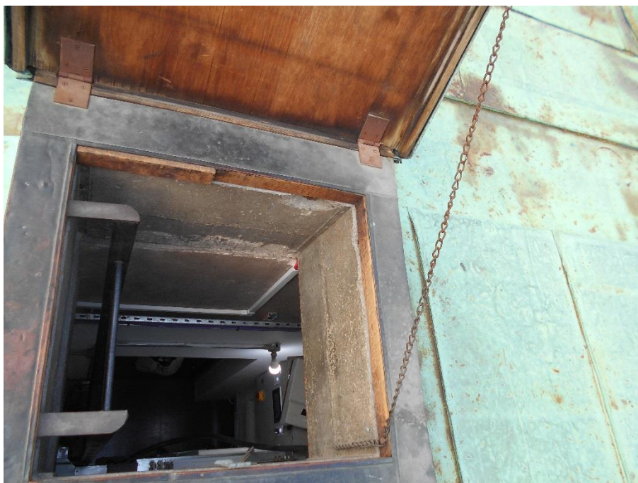
The existing roof access hatch.
