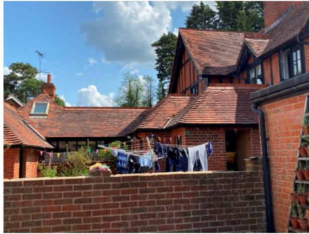
Figure 22: Extensions to the rear of Nos. 3 and 4 Kingsley Cottages
