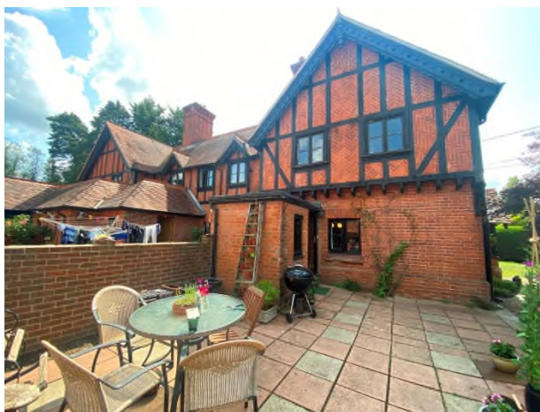
Figure 17: Rear elevation of Fielders
