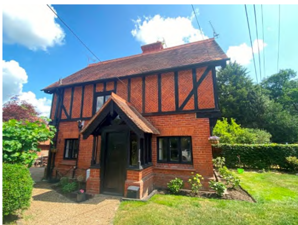
Figure 16: South-west elevation of Fielders
