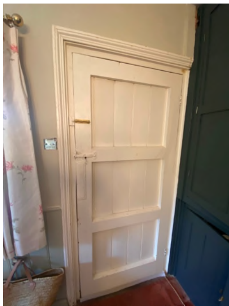
Figure 20: Rear profile of the dining room door leading to the flat roof extension
