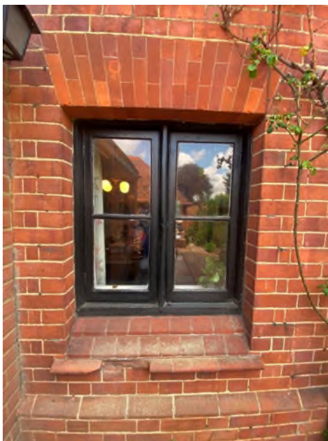
Figure 18: Ground floor window to the dining room
