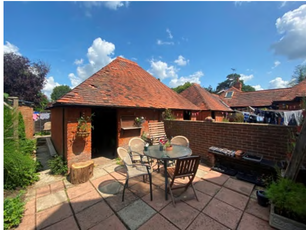
Figure 13: Brick outbuildings to the rear of Kingsley Cottages
