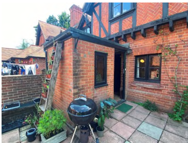
Figure 21: Flat roof extension
