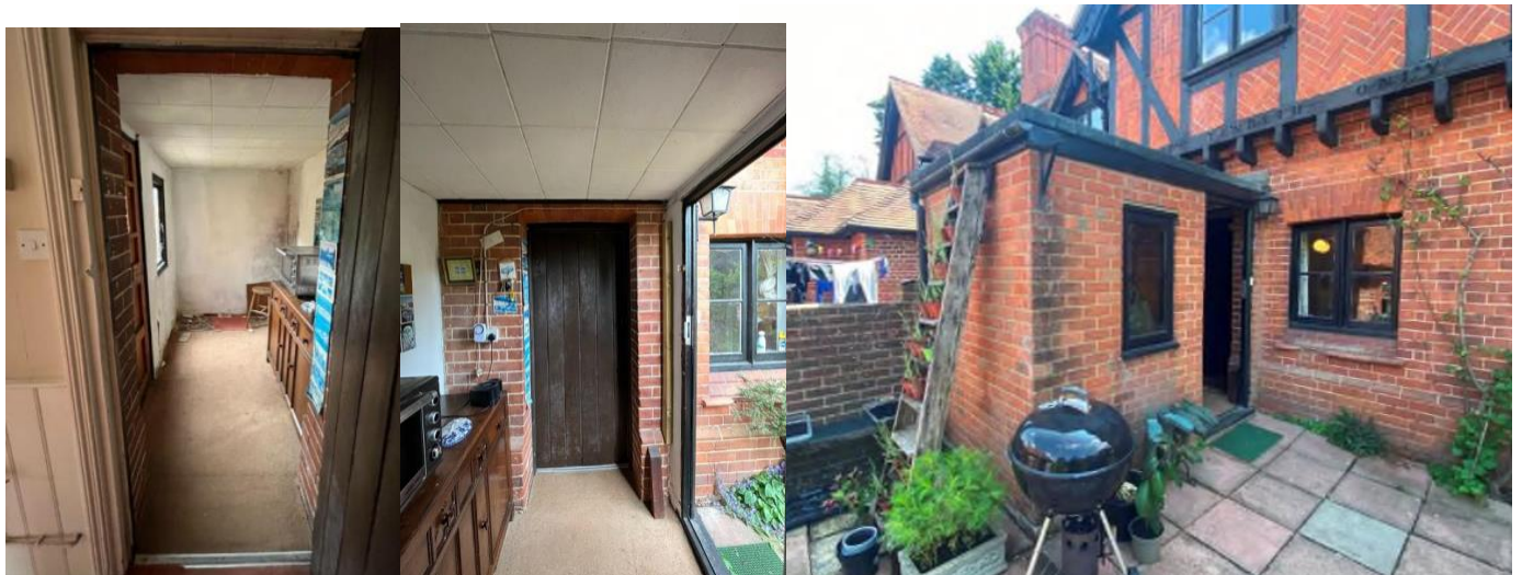
Figure 10: Existing flat roof extension (internal left and middle, external right)
