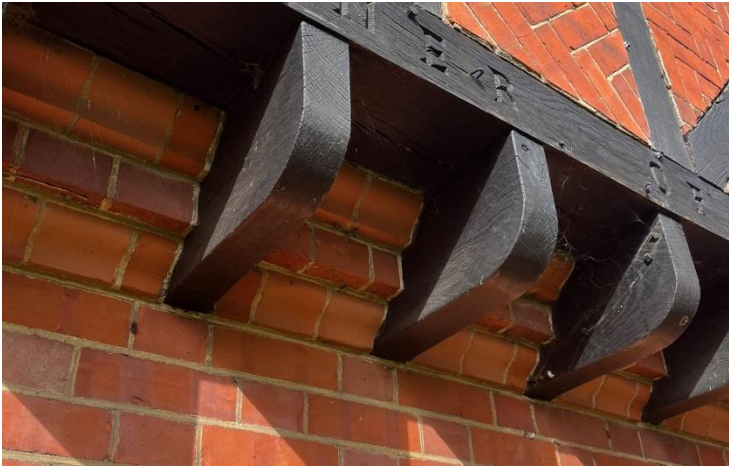
Figure 17: Photograph showing brick work under bressumer jetty on the front elevation
