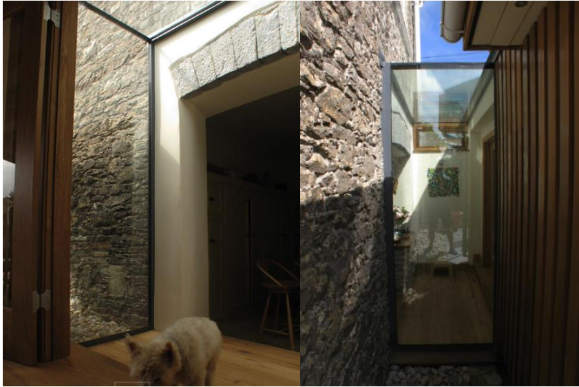
Figure 12: Examples of a structural glazed link interface
