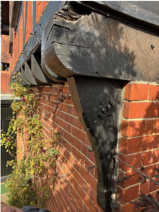
Figure 17: Photograph showing brick work under bressumer jetty on the front elevation
