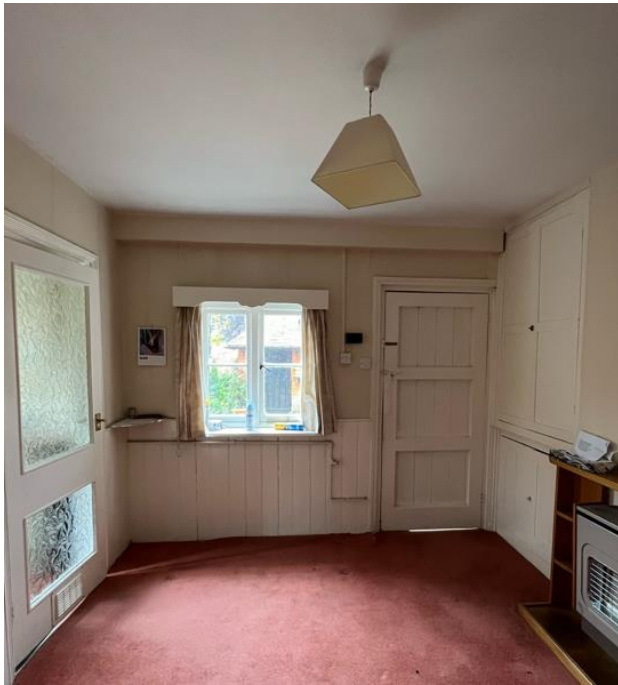
Figure 21: Photograph standing in the dining room looking towards the rear of the property with rear window and original back door.
