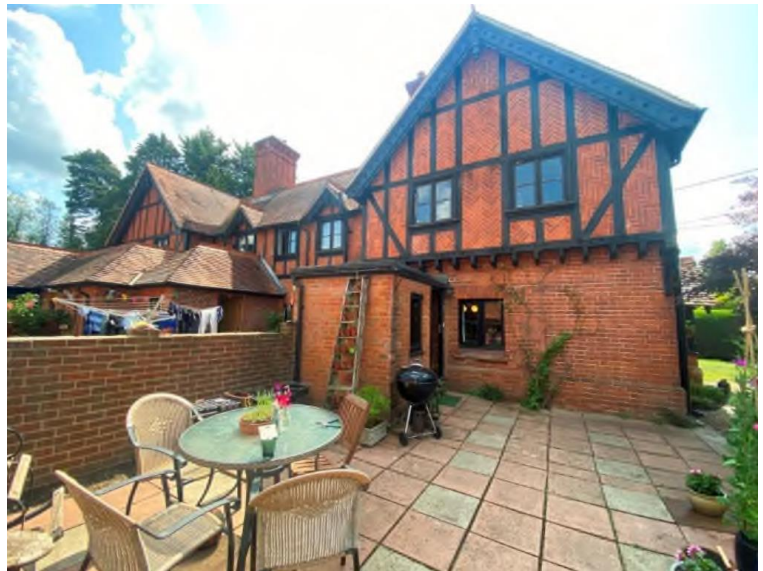
Figure 8: Rear of Fielders (North west elevation) showing existing extension and development area
