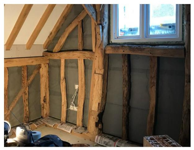
The C19 introduction of the infill first floor to the middle bay, accessed from the end bay original first floor necessitated the trimming of the original tie structural tie beam and this together with the introduction the front-facing dormer window has led to the long-term spread and distortion of the roof.
