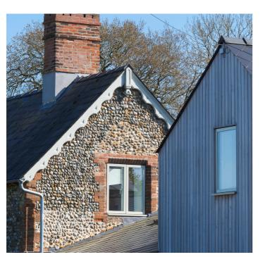
Timber frame/ aluminium cladding triple glazed windows
