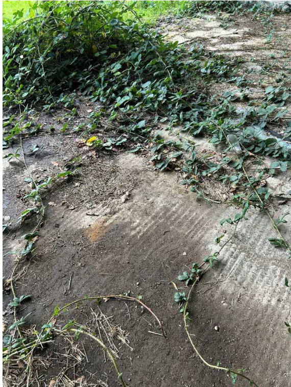
Figure 2: Existing Floor Slab
