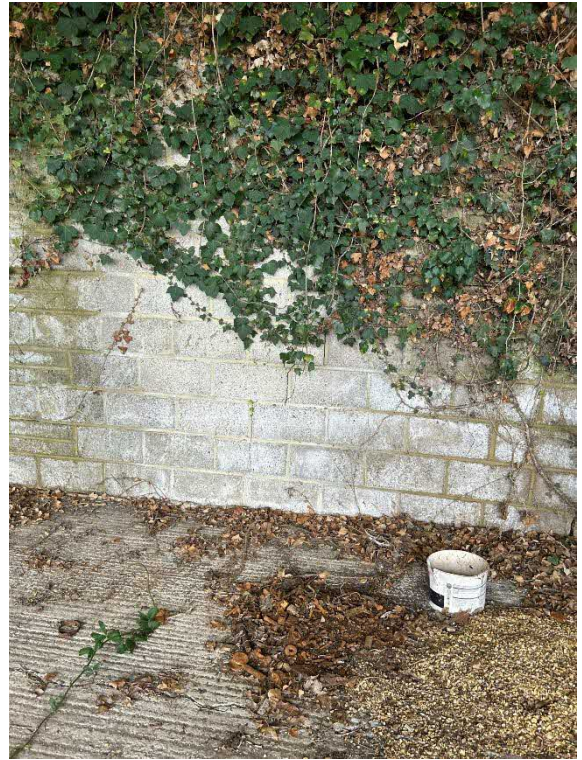
Figure 7: base of blockwork wall (internal)
