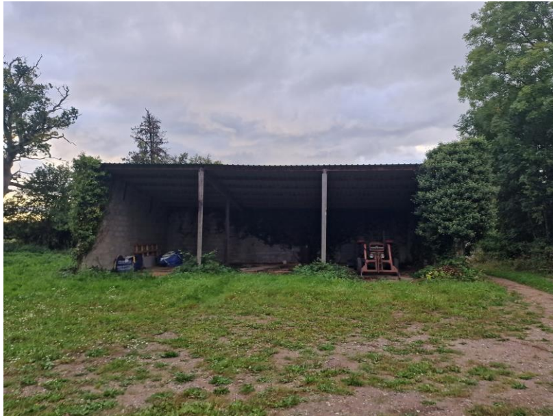
Photo 1: The front of the open barn, the south-east aspect
