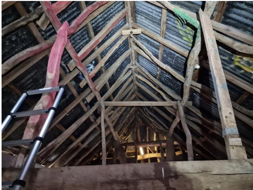
Photo 8: Internal view of the old stables showing the variety of old untreated wood used in the roof construction.
