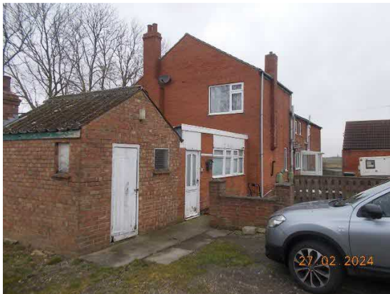
Plate 3: the residential property (Target Note 2). Photograph taken from the south-east. This house will be retained undamaged and in situ during the project.
