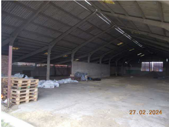
Plate 5: the interior of the large barn (Target Note 3).
