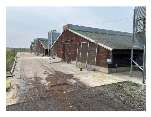
The existing buildings are of timber construction with natural ventilation.
