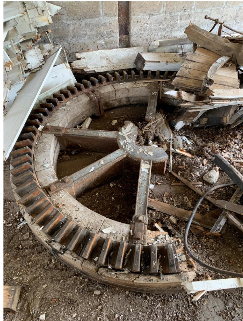
Brake wheel in current broken state following 2020 gale
