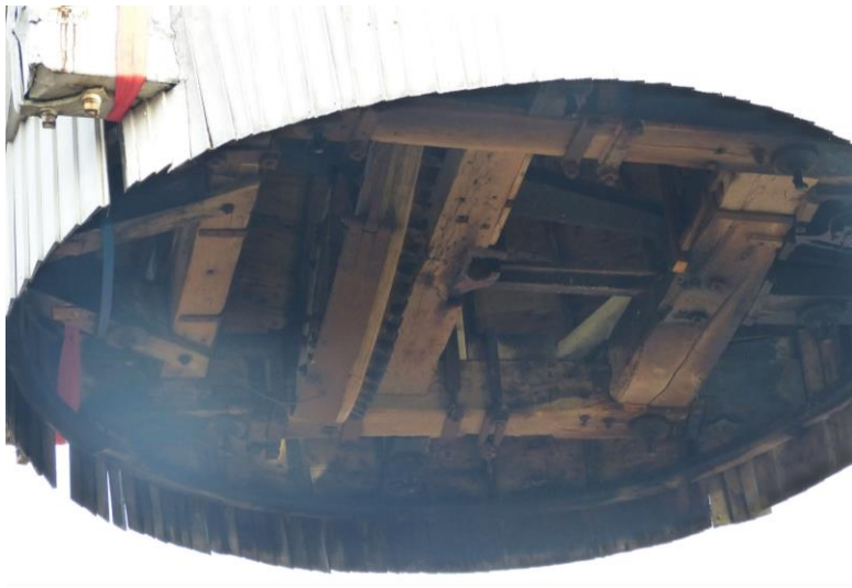
Cap underside during lifting for 2013 repairs / renewals
