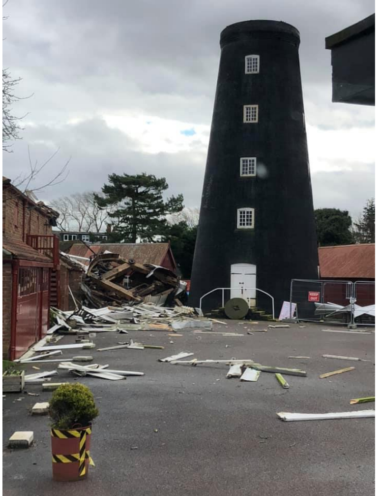
Figure 6: The decapitated windmill in February 2020, showing debris from the shattered cap and sails strewn across the yard.
