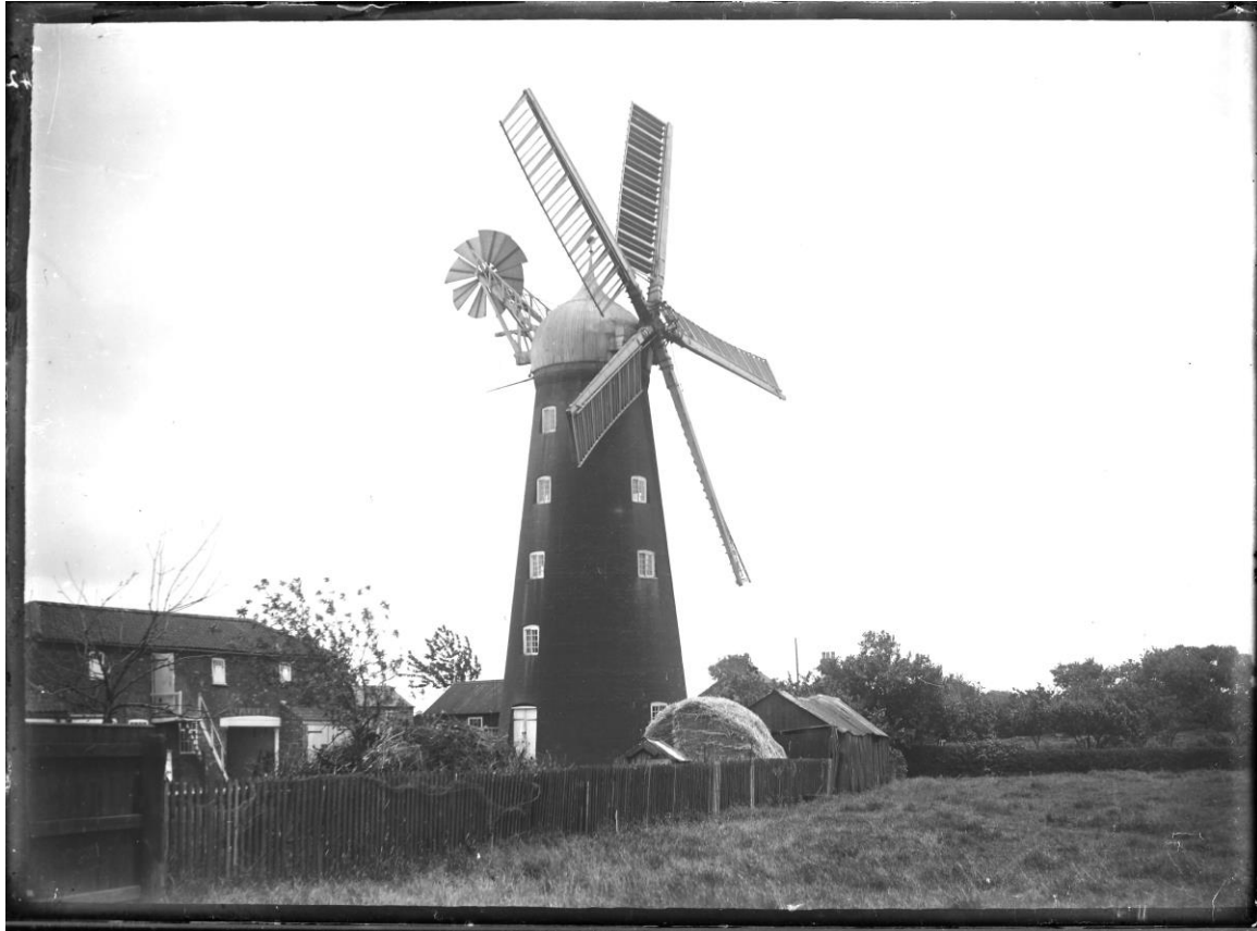
Figure 1: A glass plate negative taken circa 1935. The mill stands in a yard with outbuildings, its five sails, 'ogee' cap and eight-bladed fantail clearly visible. From the Mills Archive Rex Wailes Collection.
