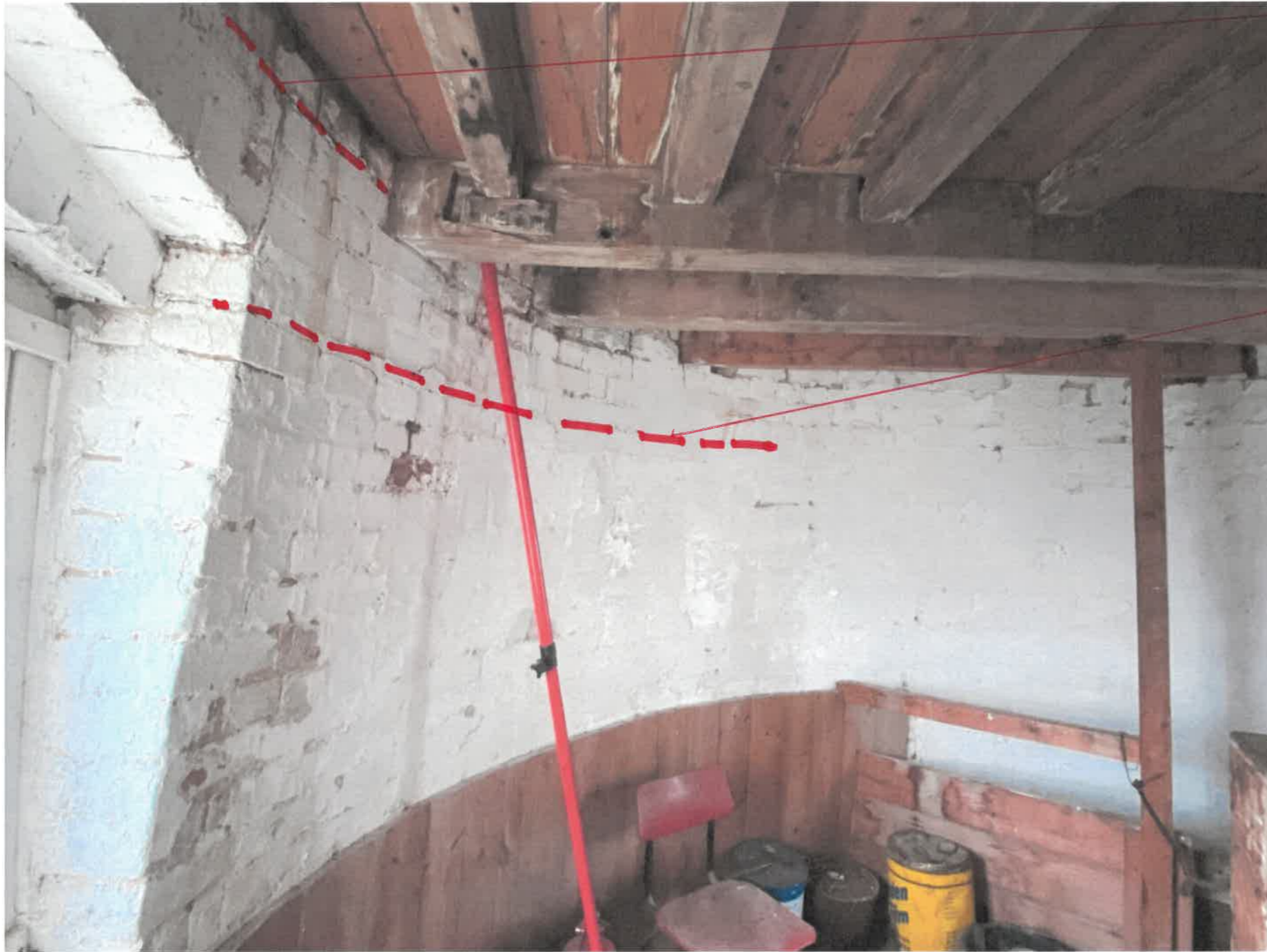
View looking south, window E4 on left
