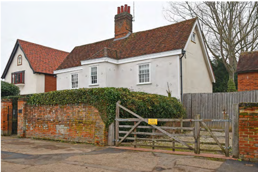
Figure 9. Front Elevation looking northwards from Church Street.
