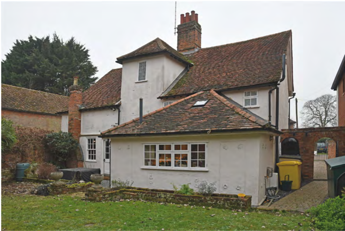
Figure 12. Rear Elevation with C20 Kitchen in the foreground. This kitchen is to be replaced by the authorised extension. There is an existing rooflight with light tube on the C20 kitchen roof.
