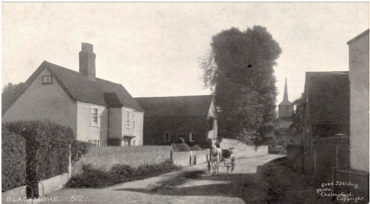
Figure 7. Photograph of Little Jericho looking south along Church Street in circa 1910. This shows that the eaves detail on the frontage was a traditional open eaves to a downpipe of the front elevation and that the render was not divided into panels. Photo: Andrew Smith.
