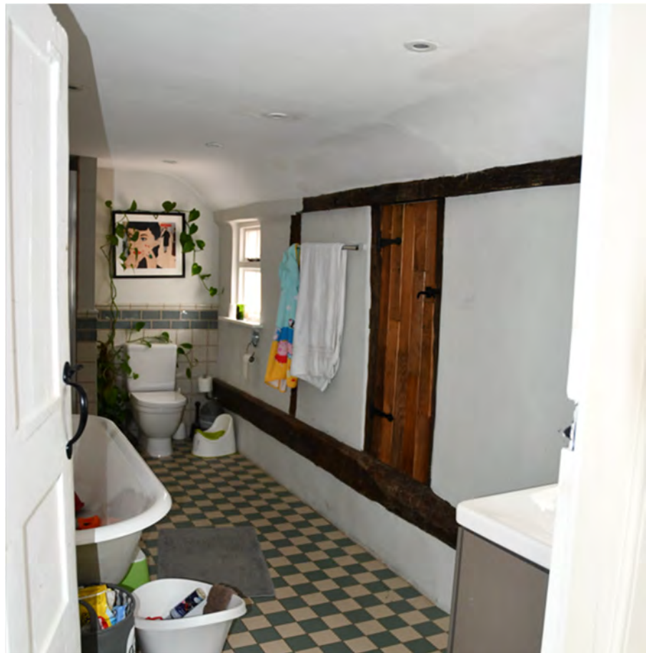
Figure 15. Existing Bathroom with substantial horizontal beam just above floor level and the two main studs.
