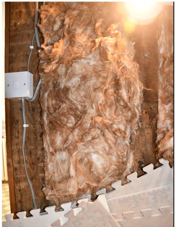
Figure 17. Detail of the historic studs showing they were originally covered with plaster.
