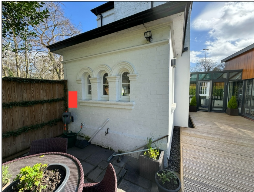
Photograph 2: Proposed location of the charging unit
