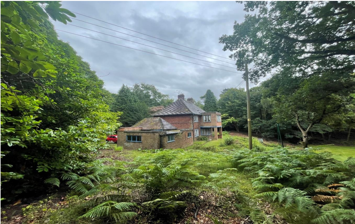
Figure 3 – View of existing property from north looking south
