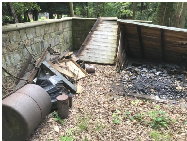
Collapsed coal shed inside terrace
