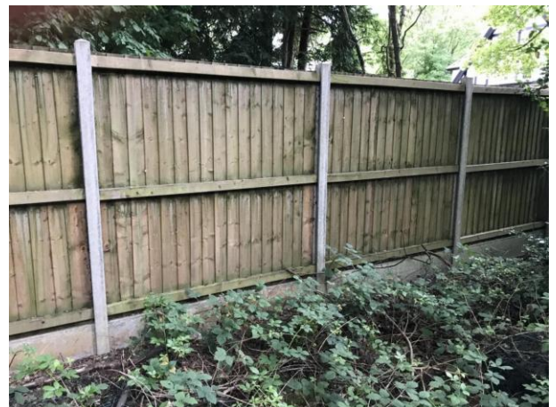
Typical boundary fence
