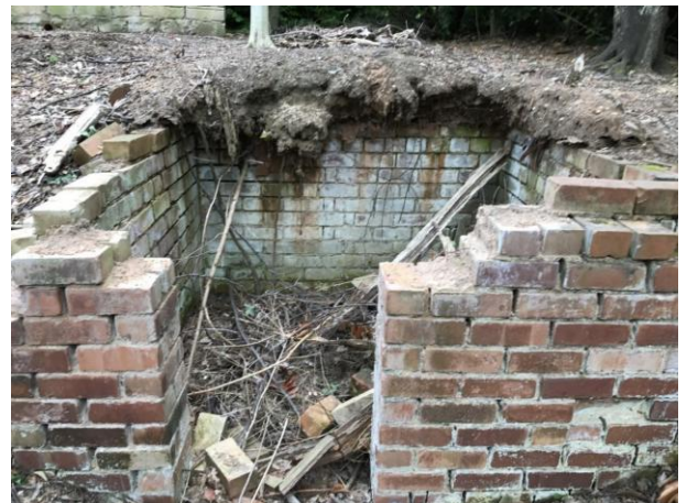
Brick foundations near terrace
