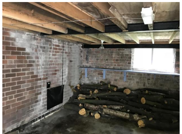
Interior of northern garage
