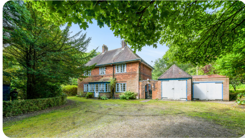
Front facade - East Elevation
