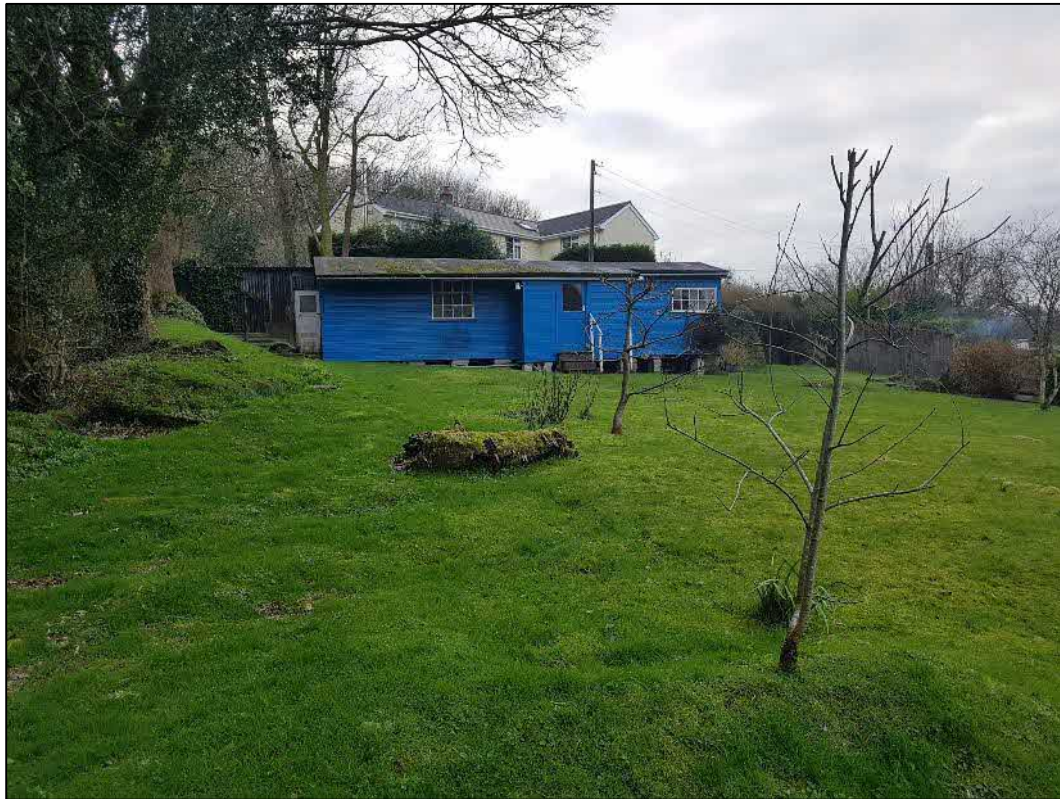
Main view of the existing building from the east.
