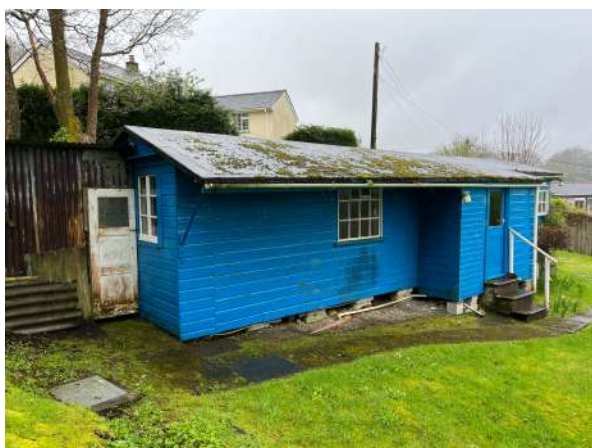
Photograph 1. South and east elevation.
