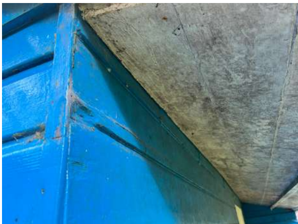
Photograph 3. Tightly fitted soffits.
