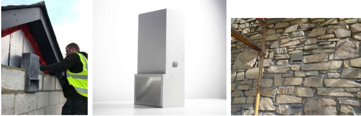
Photograph 5. 'Green and Blue' bat block and built in woodstone bat box `.
