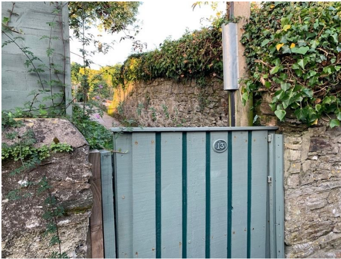
Rubblestone wall between No 13 and the proposed plot
