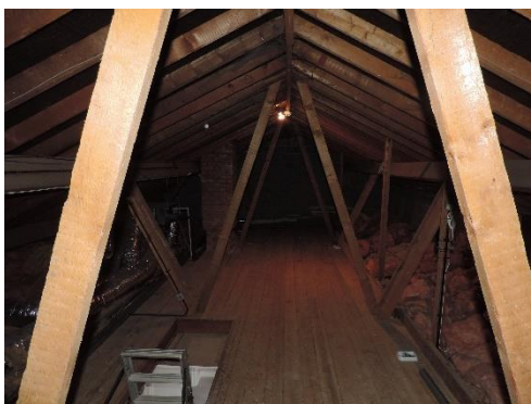
Plate 11: Birchwood Loft Space
