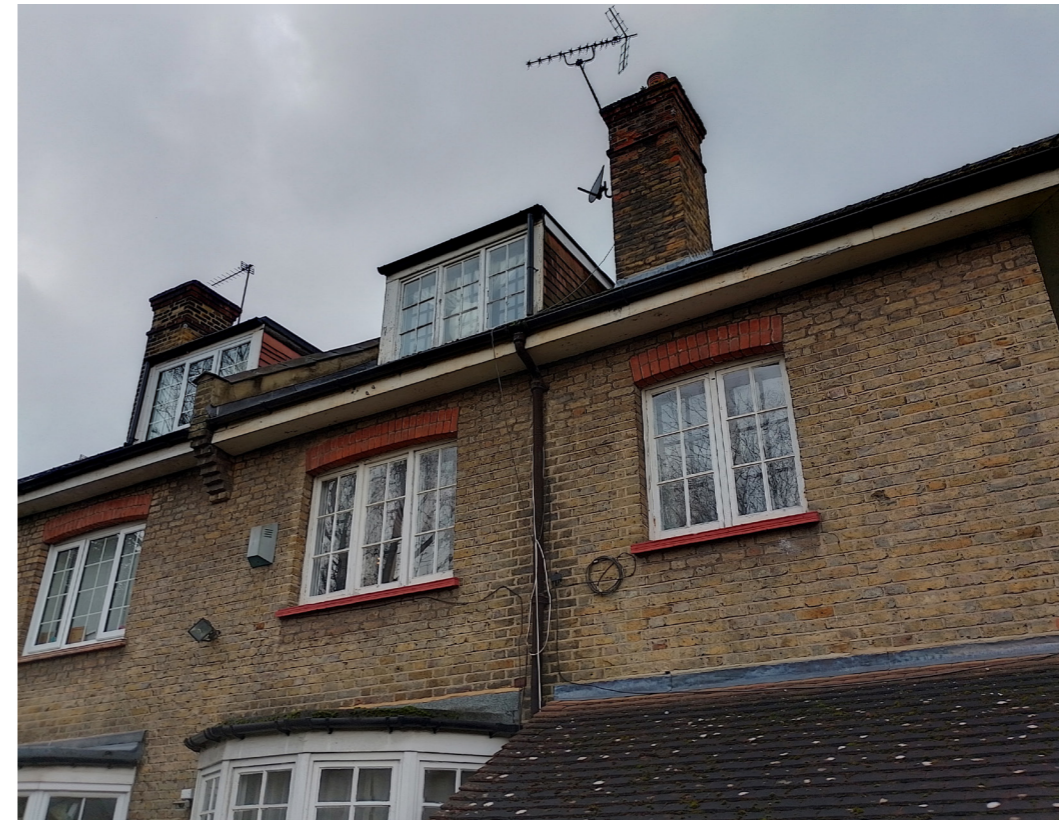
Existing brick facade detail
