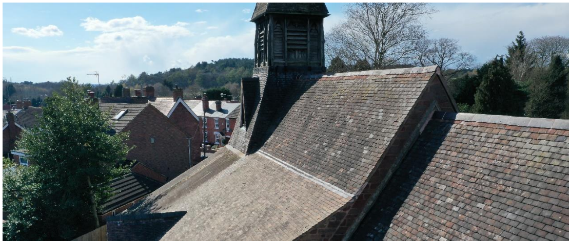
Fig 4. Photograph showing existing Bell Tower, Nave and Chancel roofs.
