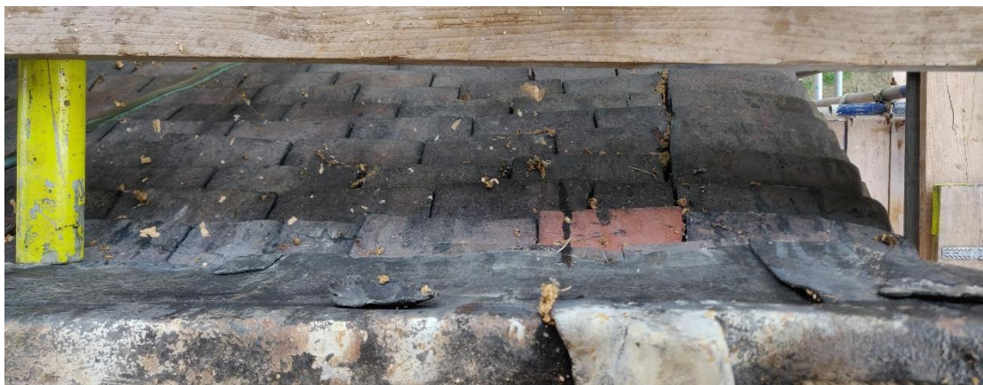
Fig 5. Photograph showing existing bonnet hip detail and top cover flashing.
