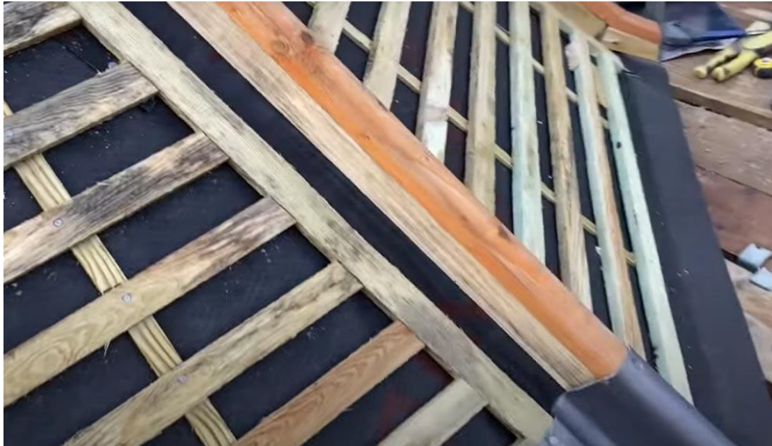
Fig 8. Photograph to illustrate the proposed lead-roll hip detail.
